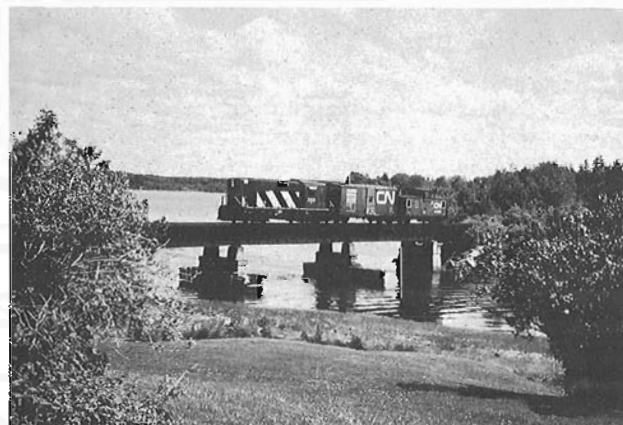
Picture 1 (one). Eastbound freight train on French River bridge.
