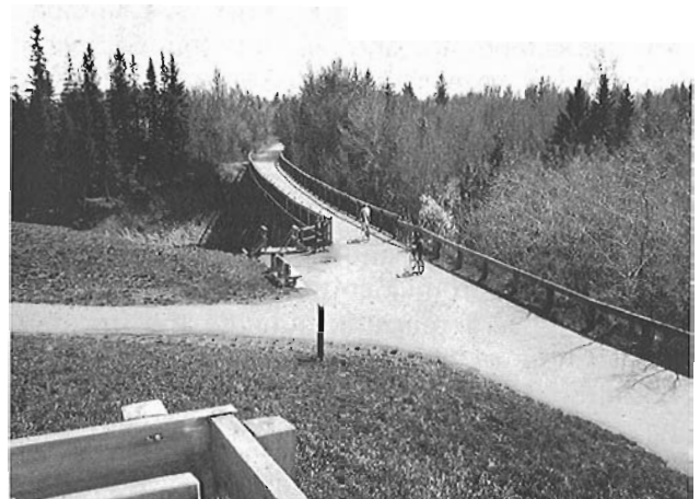
All the old trestles were left as they were, but there's fenced railing along the sides for safety.
