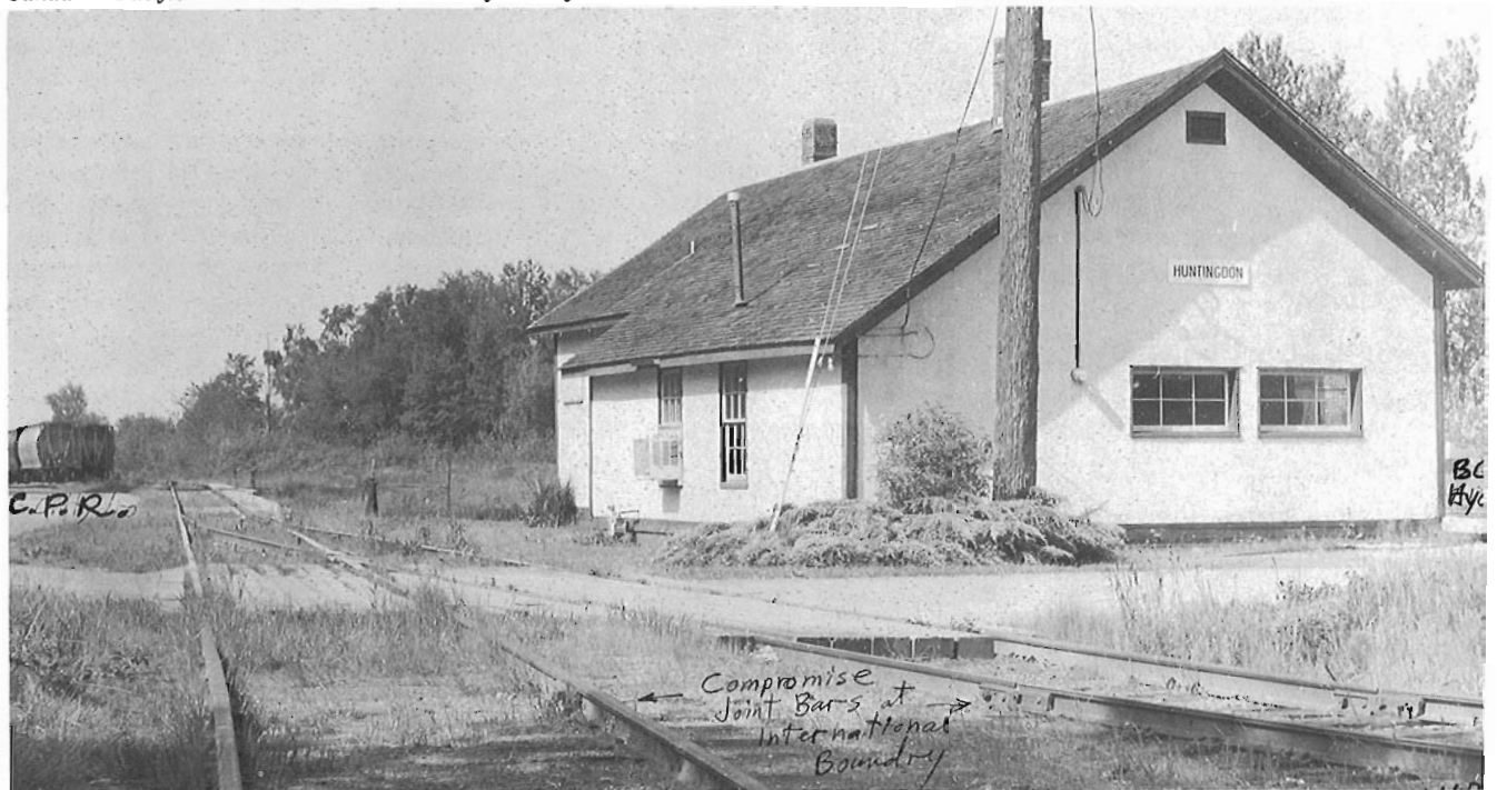
Then Ed. Wilkomen strolled back into his own country and shot a view into Canada. Note that at the exact border the tracks (MILW on the left and N.P. on the right) have compromise joint bars on them. This is because Canadian Pacific likes to use larger size rail.
