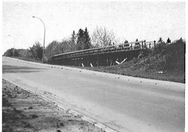
Another view of the old trestle alongside 76 Ave. looking west.
