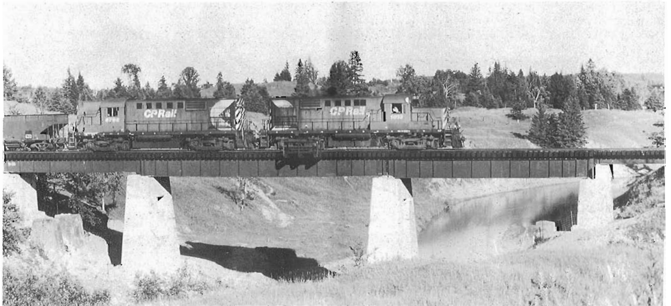
C. P. 1813 (ex-8765) and 8796 cross the bridge westbound over the Quyon River on July 21 1986 (the 150th anniversary of Canadian Railways). Note the old concrete piers from an early bridge likely replaced when the mine was opened in the early 1950's.
