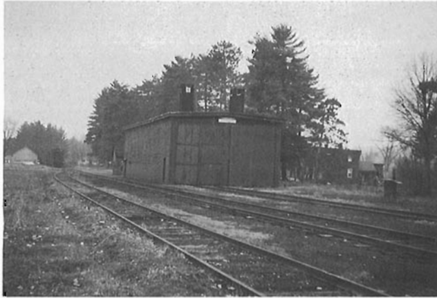
The two-stall engine shed at Waltham Que. as it appeared in 1965 shortly before it was demolished. Photo by Bruce Ballantyne.
