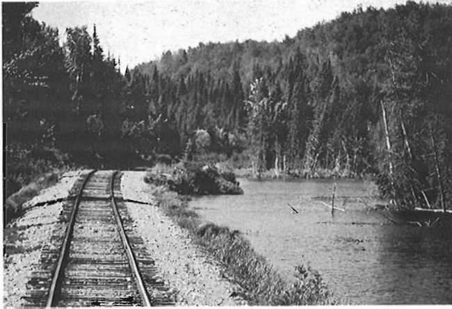
Scene along the right-of-way on the Thurso Railway at mile 31 looking south.
