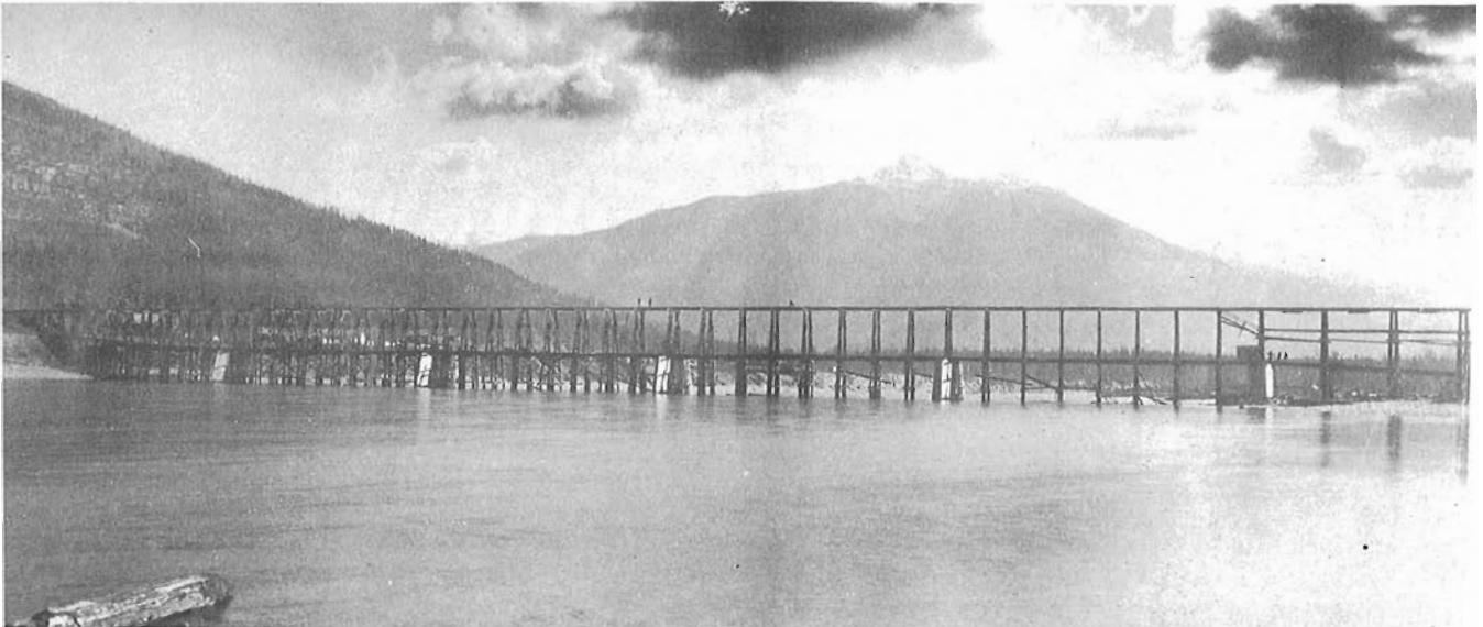
Temporary trestle on the Canadian Pacific Ry main line over the Columbia River at Farwell, later Revelstoke, B. C. 1885.
