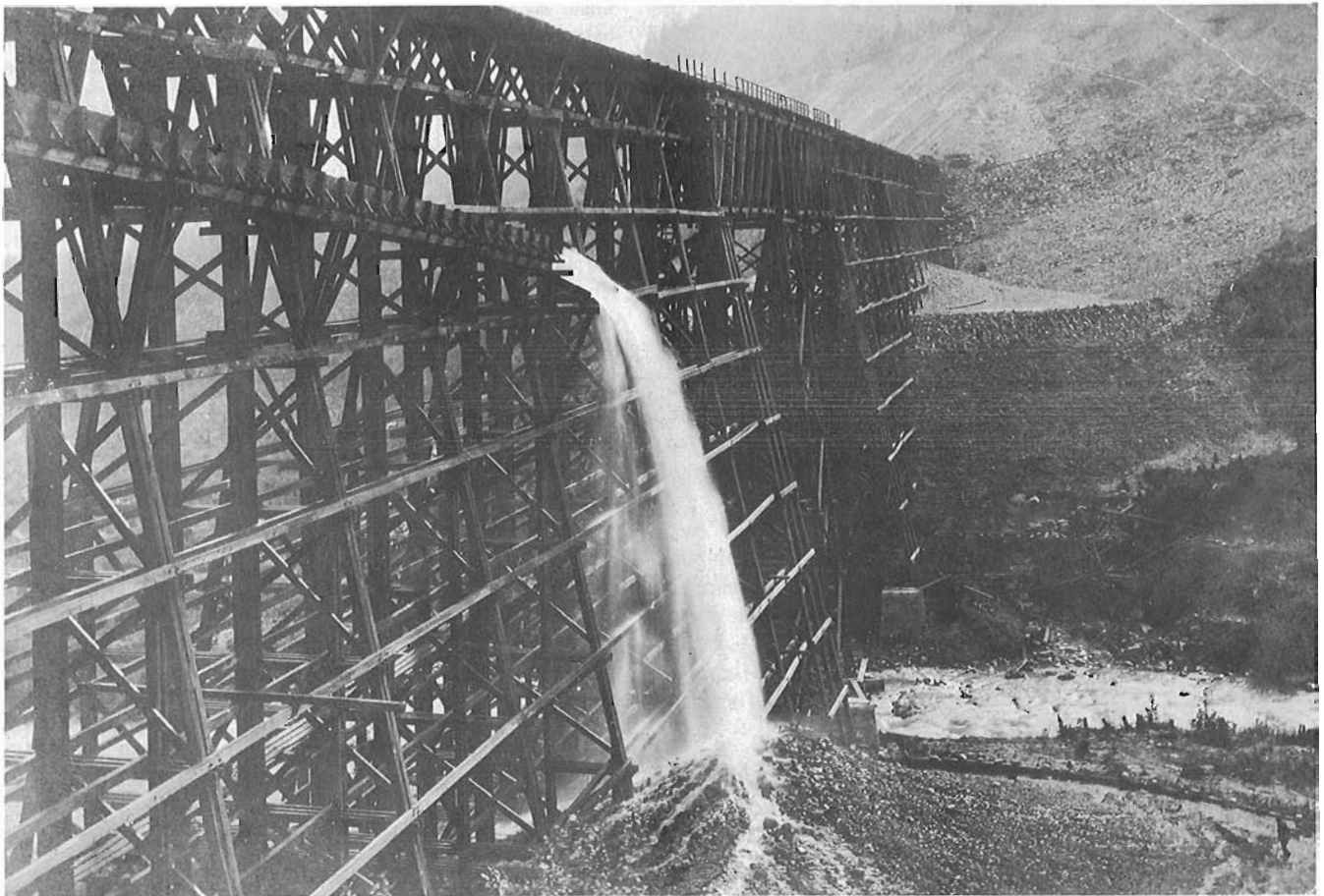
The disappearance of the large wooden trestles constructed during the mid 1880's took many years to effect. In 1897, CP started to fill in the Mountain Creek trestle using sluices and flumes to bring down gravel from a source above the trestle. The cost of this method was reported as one half that of using conventional method of bringing the fill in by trainloads. Filling in the trestle took four work seasons and some 300,000 cubic yards of gravel.
