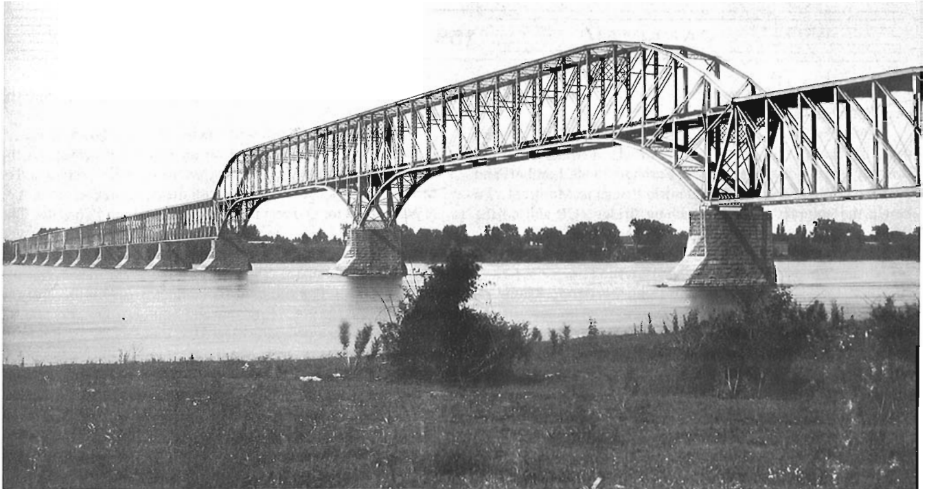
Canadian Pacific Ry St. Lawrence River bridge, viewed from the south-east. November 7, 1901.
