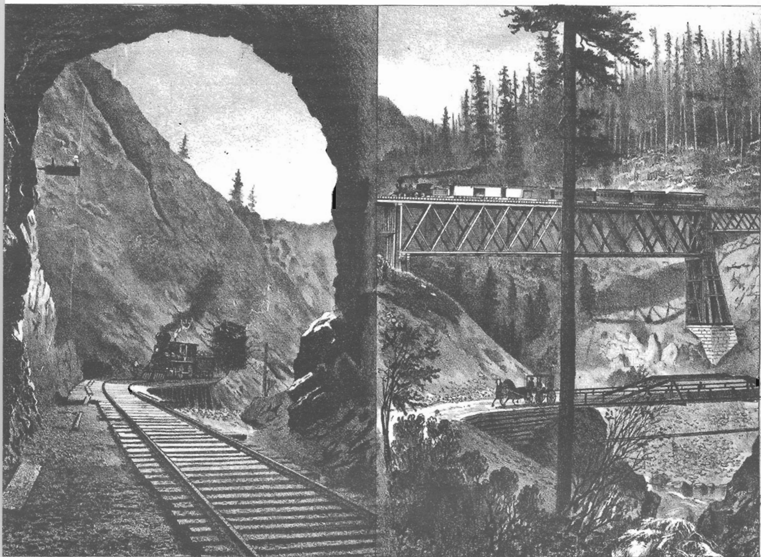
• LOOKING WEST FROM TUNNEL 3 INTO 2 •
