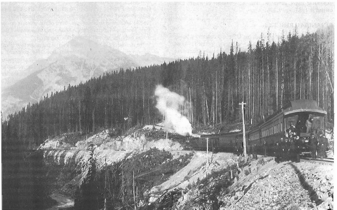
The "Pacific Express" on the Big Hill circa 1888. Above the locomotive and the mail-express-baggage car may be seen one of the run away tracks built as a safety measure to stop any trains which may have lost their brakes on the hill.
