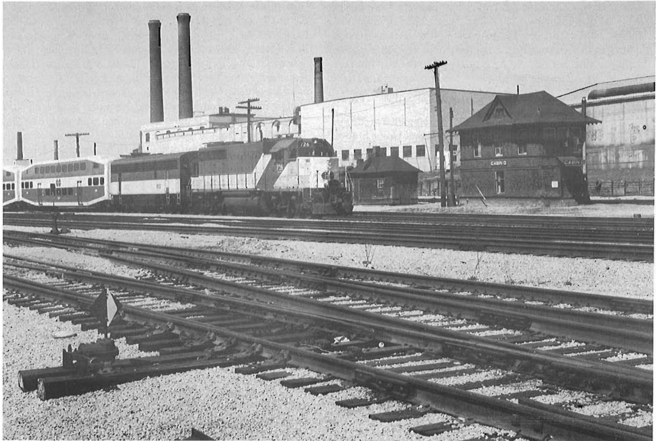
Prior to the completion of the flying junction and CTC signals, movements through the interlocking at Bathurst Street were controlled from Cabin D. In this September 1985 view, a GO Transit train enroute to Union Station passes this venerable structure. Both units heading up this train came from the United States. GP40 #726 was purchased from the Rock Island and APU #800, which was purchased from the Burlington Northern, was originally purchased by the Northern Pacific in 1950.
