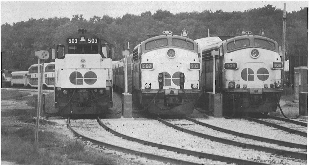
The three daily Toronto-Milton GO trains layover at Guelph Junction. In this August 1986 view are two generations of diesel power. GP40TC #503 is one of the 8 original locomotives bought for the start-up of GO in 1966. APU's 902 and 906, converted from FP7A's, were originally purchased by the Ontario Northland in 1952. On GO Transit, these units serve as auxiliary power cars to generate the electricity to operate the services on the coaches, and as control cabs for push-pull operation.
