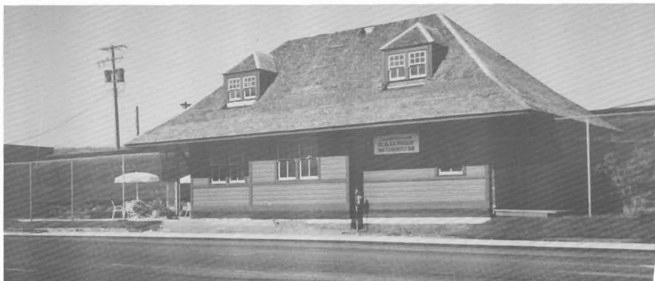
At Cranbrook, the station as viewed from the street side. Only the chimney remains to be installed.
