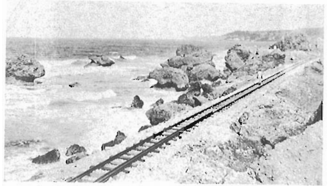
A straight section of line along the East (Atlantic) Coast, this portion of the railway was subject to vicious erosion throughout its life. Photo courtesy BMHS.
