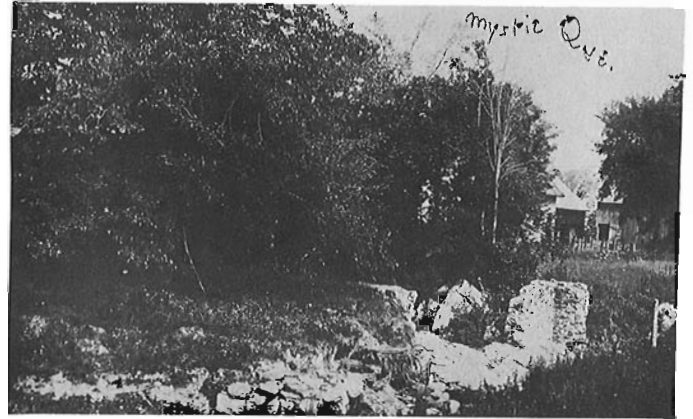
The stone corners are those of a mill, powered by water in the Mystic brook, that made roofing shingles from cedar logs grown in the area. Water held by a dam overflowed over a rock ledge on the left.
