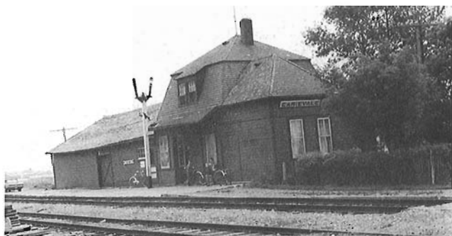
Designed by R.B. Pratt, the CP depot at Carievale Sask. was of a type flexible enough to be used on two sizes of stations as well as section houses. Only two of these were in Saskatchewan, with twenty others in other western provinces.
