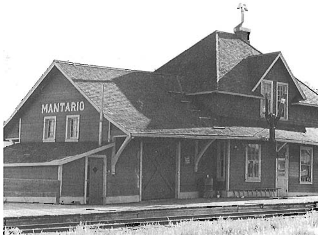
CN depot at Mantario Sask. as photographed by Charles W. Bohi in 1971. A Canadian Northern "Third Class" type, this station was built by Canadian National in 1920, and, unlike many, never had stucco applied.
