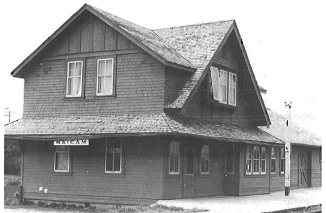
The CP depot at Naicam Sask. built in 1922, is typical of the more than 35 type "A3" stations built by CP in Saskatchewan between 1919 and 1929.
