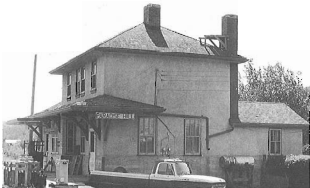
The Canadian National "Third Class" station at Paradise Hill Sask., was duplicated at as many as forty other locations in that province. By 1973, when the photo was taken, most merchandise came to the depot by truck.
