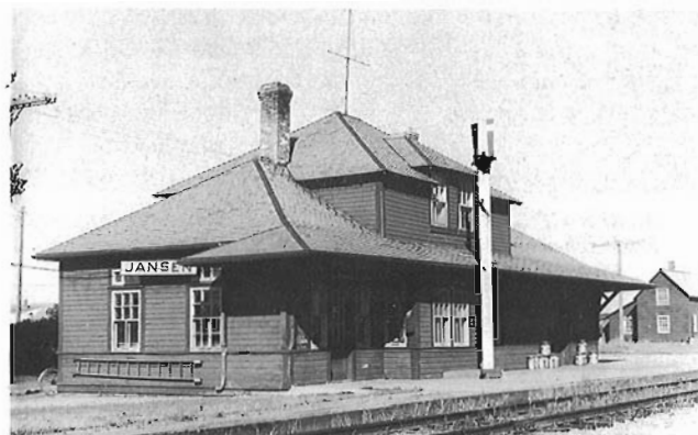
Jansen Sask. a CP "Standard Number Five" station built in 1909 and photographed in 1971. A total of 84 similar stations were located on CP lines in Saskatchewan.
