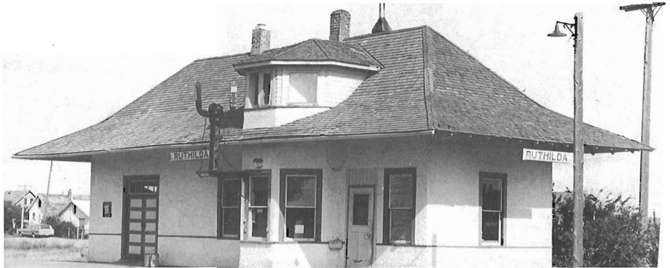
Ruthilda Sask. is typical of the 108 depots built in Saskatchewan between 1910 and 1914 by the Grand Trunk Pacific. Originally wooden sided, this station had stucco added by Canadian National. Photo by Charles W. Bohi, 1972.
