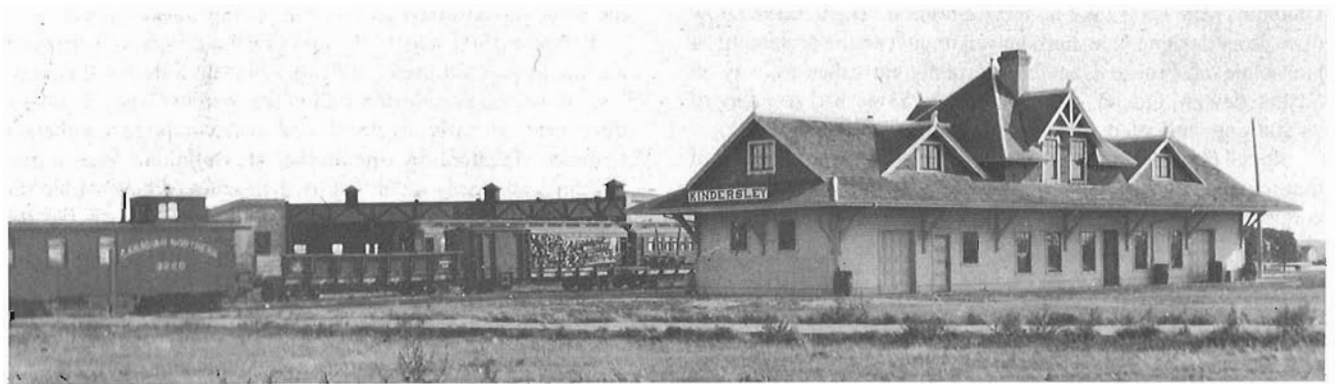
Canadian Northern built larger "Second Class" stations at Divisional points like Kindersley Sask. This station, photographed in 1913, had gone by 1972. Saskatchewan Archives Board. Photo R-A9376 (1).
