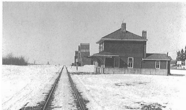
The CN "Third Class" station at Rabbit Lake Sask., was on the same side of the track as the grain elevators. This was a new layout, designed for safety reasons around 1910. This station never had stucco applied.
