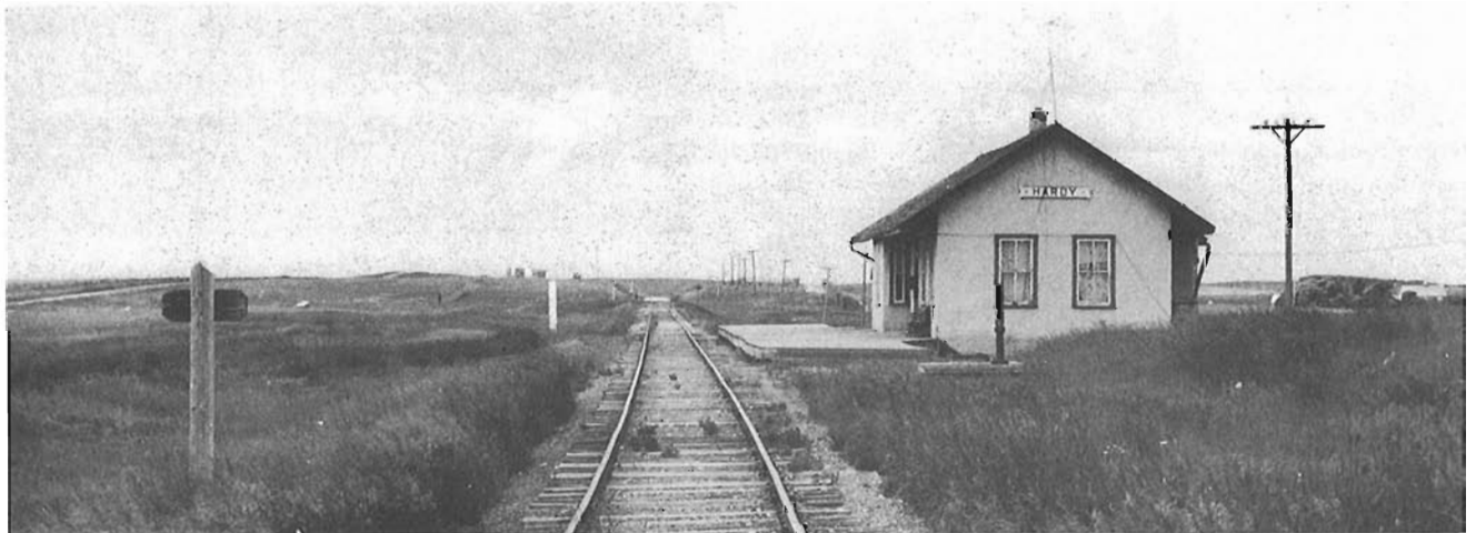
The Canadian Northern station at Hardy Sask. is a "Fourth Class" depot built in 1918 at a time when Canadian Northern's grand visions had been destroyed by its financial difficulties. Photo by Charles W. Bohi, 1970.
