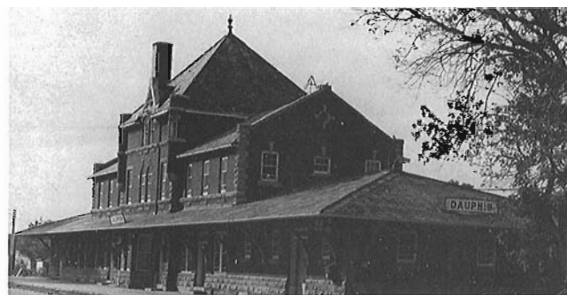
The Pratt roofline was so versatile that even large stations like this one at Dauphin Man. had them. A similar station once existed at Saskatoon Sask.
