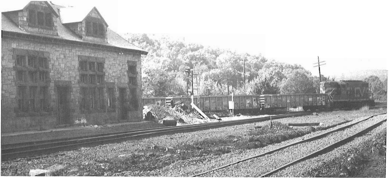
An Amtrak work train, hauled by CV locomotive 4923, at Palmer, Mass. during the rehabilitation of the future route of the Montrealer, in September 1988.
