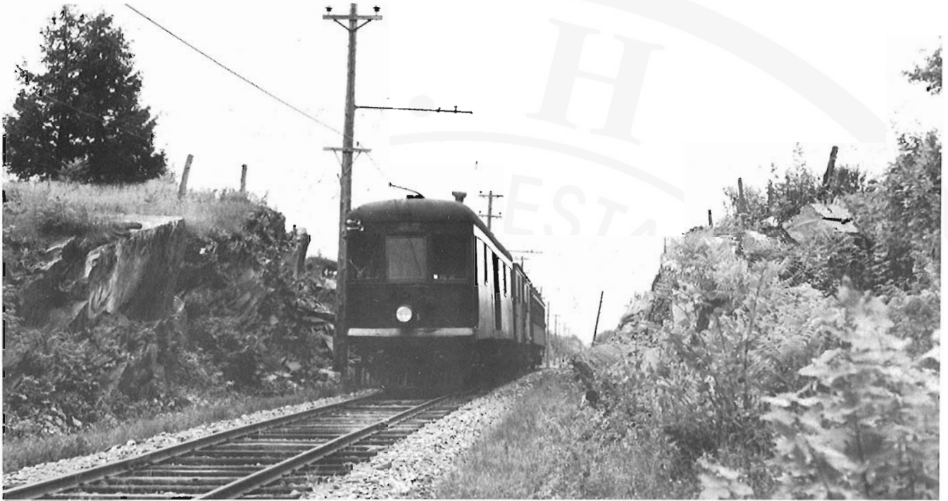
An interurban train passes through the rock cut near Abbotsford Que. on August 4, 1951. CRHA Archives. Toohey Collection. Photo 51-627.
