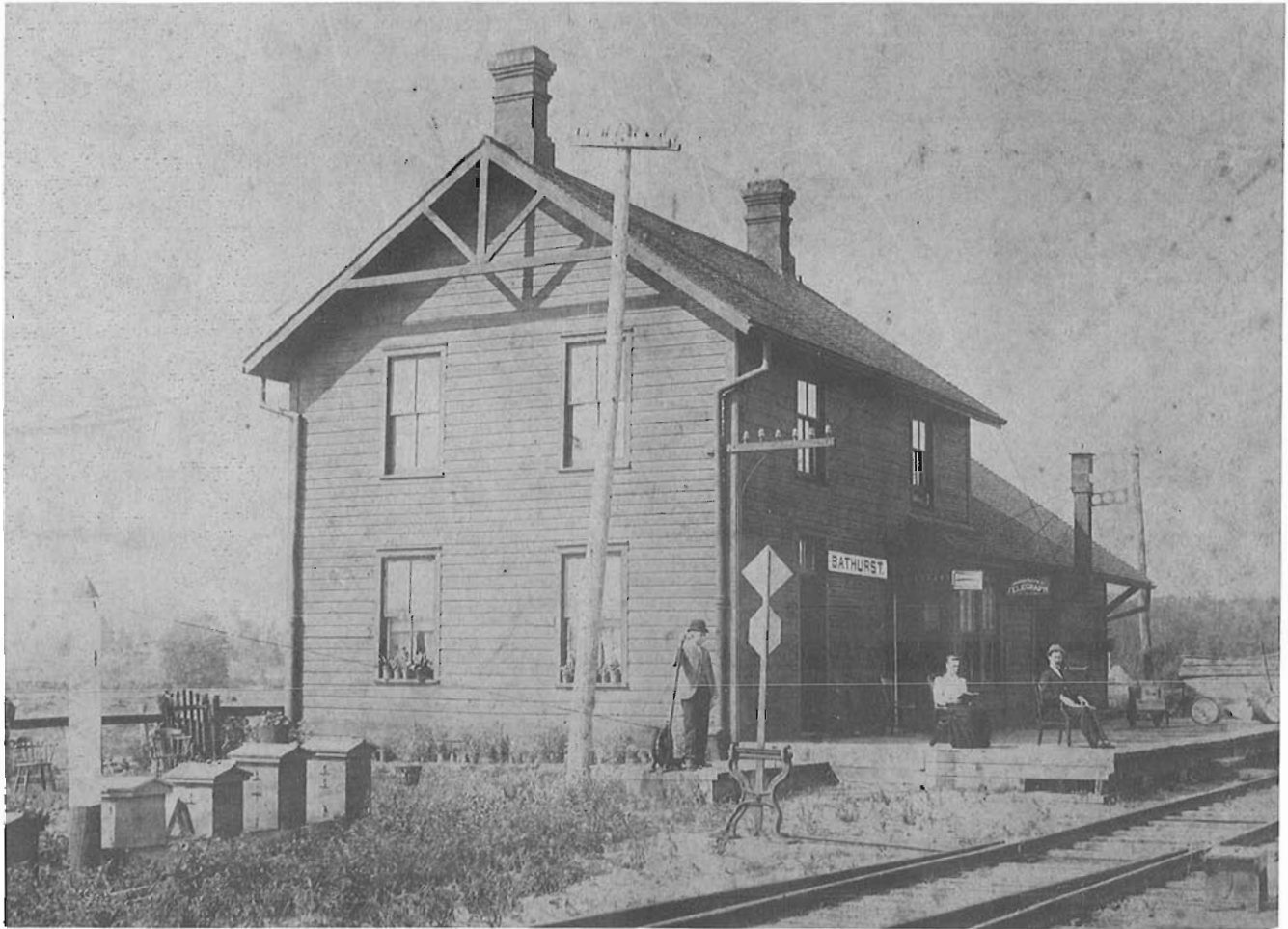
Bathurst, Ontario eight miles west of Perth on CPR's (nee O & Q) mainline in the mid-1880s. My grandparents are seated on the platform and great Uncle stands beside a signal winch. Note the Dominion Express and Canadian Pacific Telegraphs signs, a weight scale, station house signal, fire buckets, platform pedestal and especially the switch standard and tracks.
