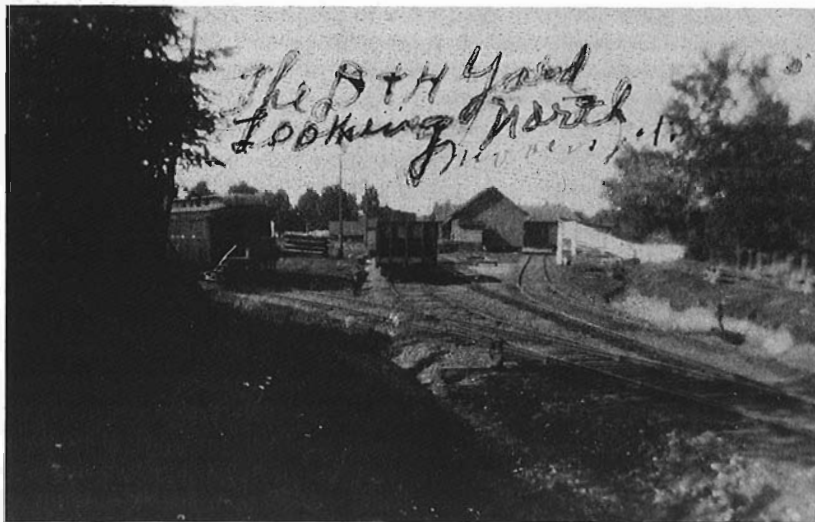
The D. & H. yard looking north. Note the ancient coach used in work service.
