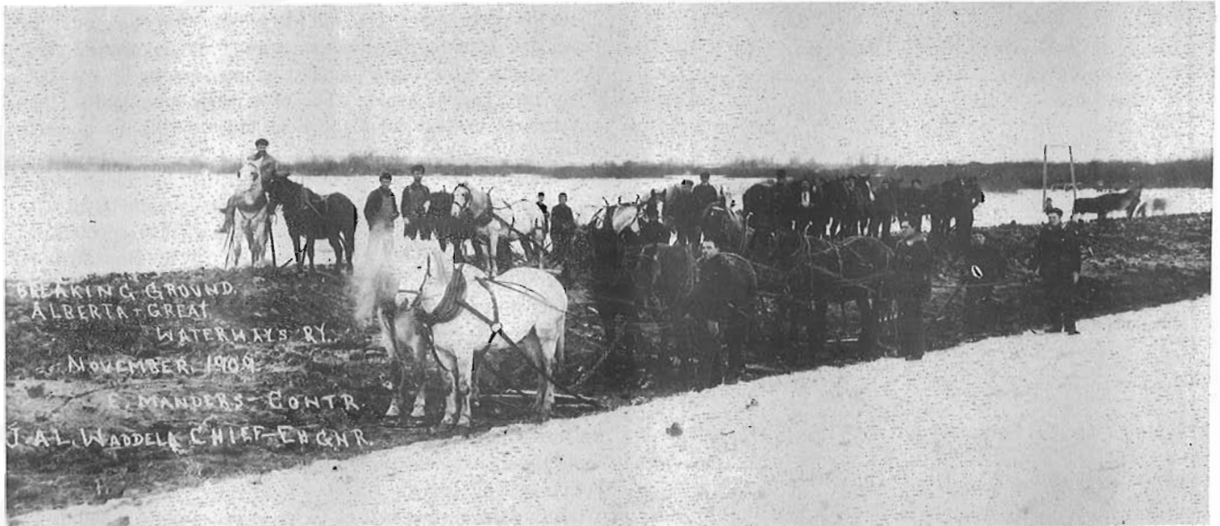
Contractor Manders and his men break ground on the Alberta and Great Waterways Railway in November 1909.
