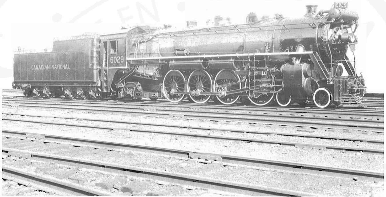
The Early 6000' s. A brand new U-1-b , 6029, built in 1924. One of my favourite types of Canadian National locomotives fondly remembered as the power on the Continental Limited. C.N photo 23126.
