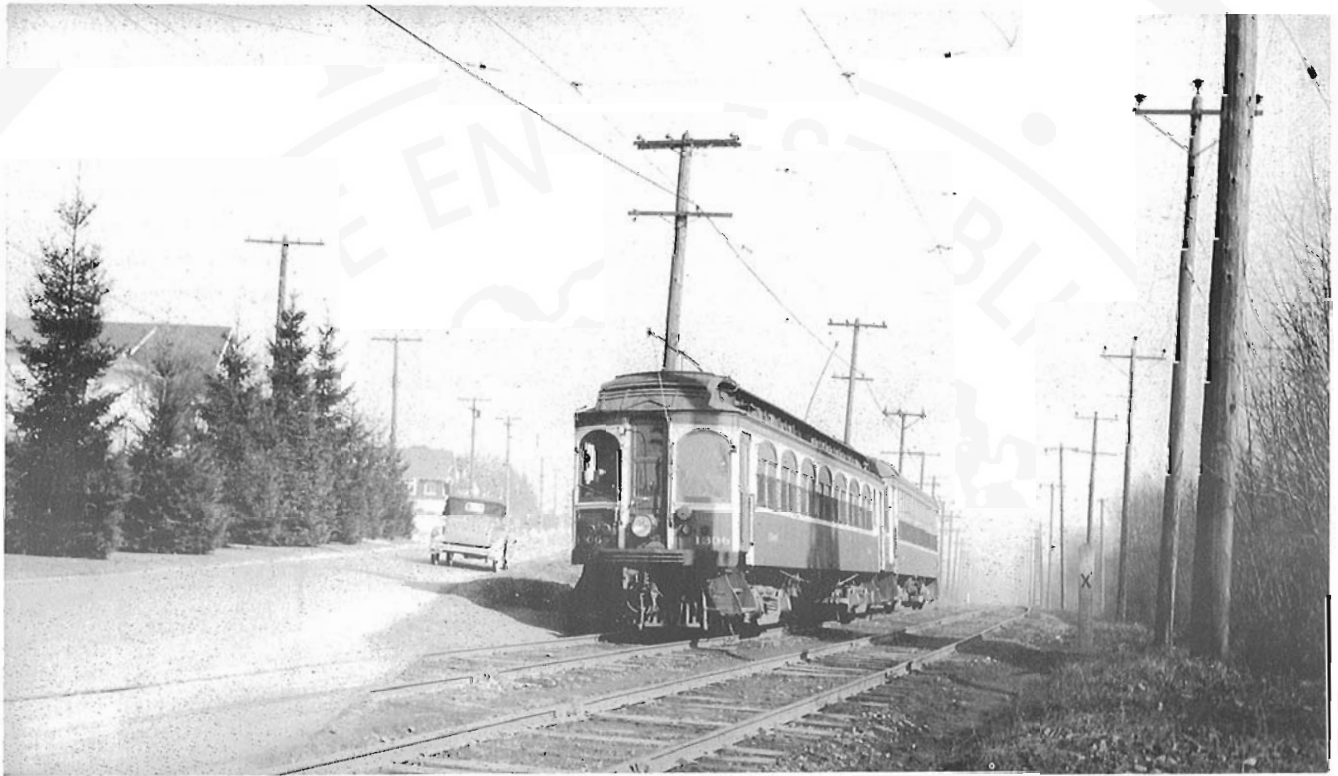
Filled with Vancouver-bound commuters, a Central Park line train ascends the Highland Park cut-off, led by 1306, one of three B.C. Electric Kuhlman products of 1911. The other car in the train is one of the twenty-eight interurban coaches received in 1913 from the St. Louis Cuy Company. Henry Ewert collection.
