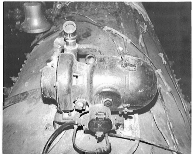
The turbo generator, which produces electricity needed for the lights etc. on the locomotive, sits atop the boiler.
