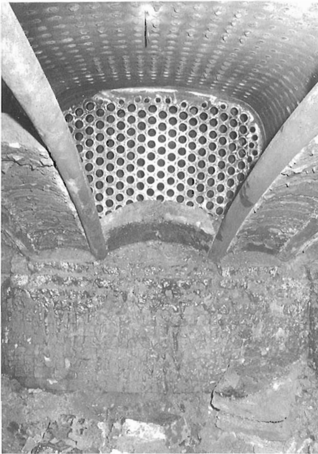
Arch or siphon tubes, and rear tube sheet.
