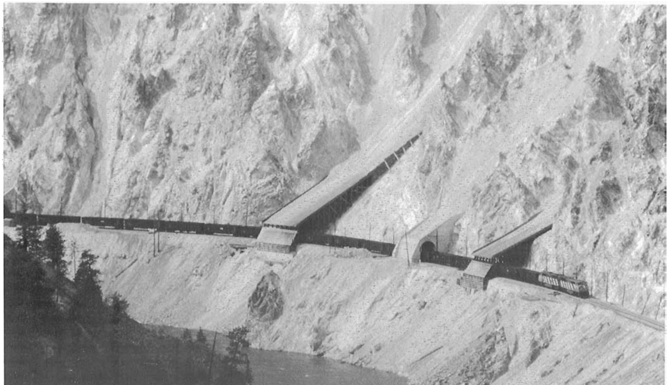
Immediately north of Lytton, B.C., the CN line runs along the stupendous gorge of the Thompson River. In order to prevent rock and snow slides from blocking the line, CN has built a number of sheds to protect their trackage. In this May 1986 view, an empty CN coal train is proceeding westward to pick up yet another load of coal.
