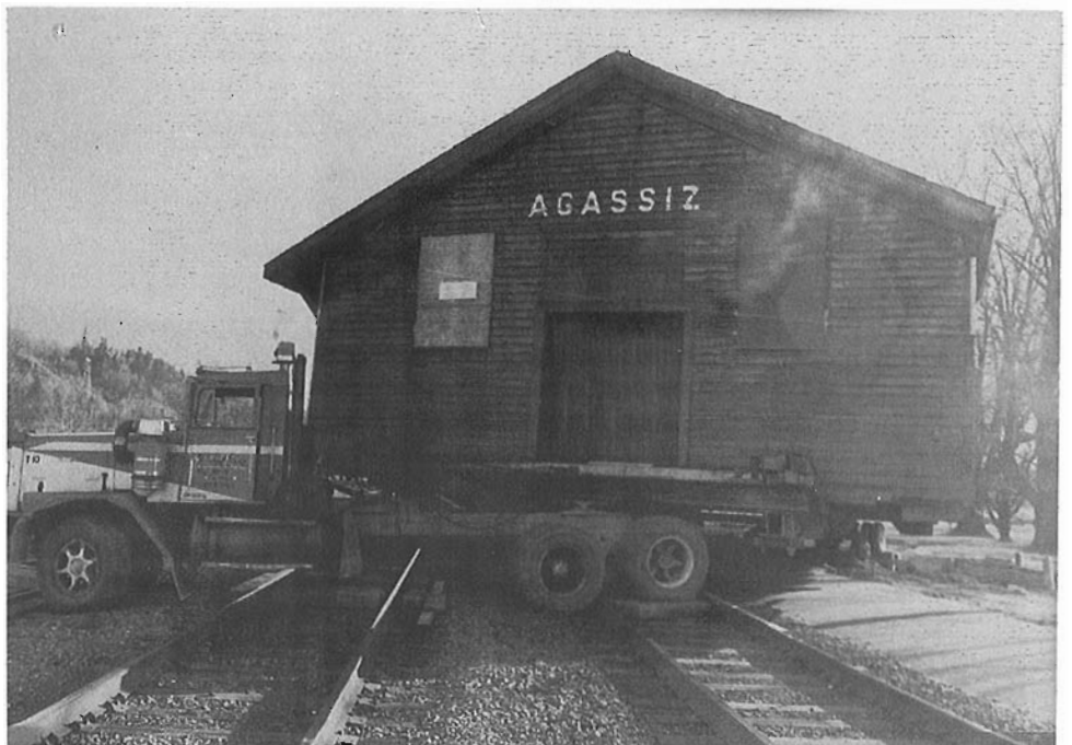
One of the major parts of moving the station was crossing the main line C.P. tracks.
