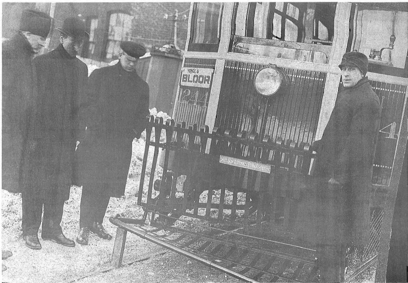
The Watson Automatic Fender, 1908 Type. Showing Flexibility. Conforms to condition of road bed.
