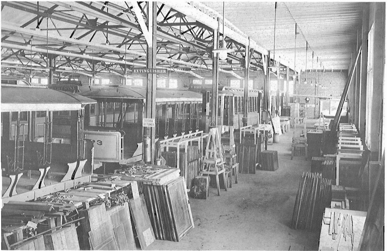
Rebuilding 651-class double-truck open cars into closed PAYE trams in 1912. Car 673 in the foreground is about to be started, while 687 in the background is almost complete, and already has its PAYE number panel. This photo was taken in Youville Shops soon after they were opened, and it shows much detail as well as some cars of older and newer types.
