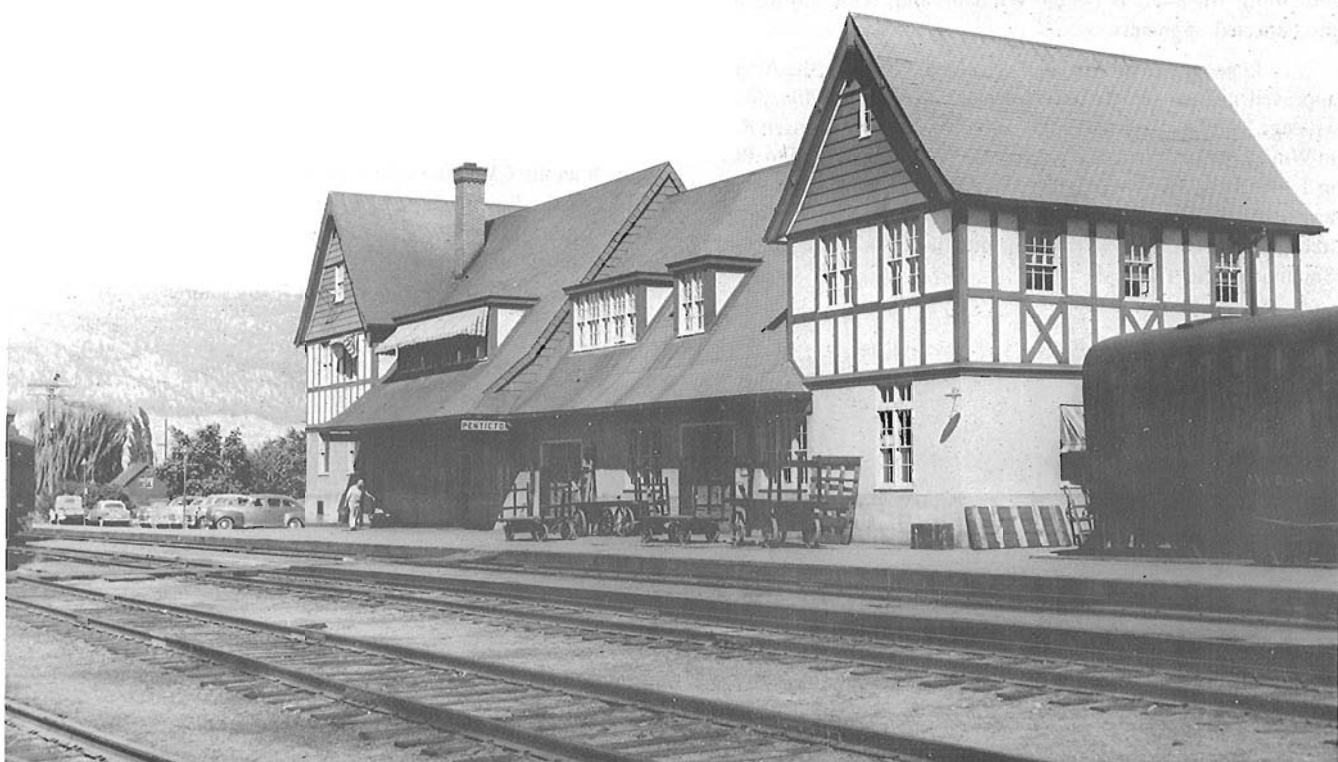
On December 12, 1941, CP opened a new combined station-divisional office building at Penticton. After the war, an extension was built on the eastern end bringing the structure up to the size shown in this photograph taken on August 30, 1952.
