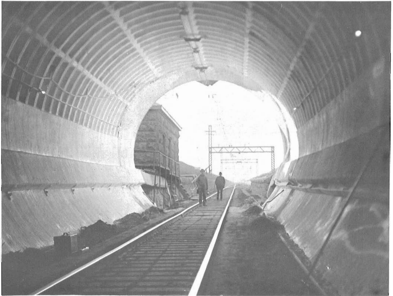
ABOVE. On November 9, 1908, photographer John Boyd recorded this view of the renovated interior of the tunnel. This view which looks toward Port Huron, Michigan shows the heavy catenary supports adopted by the GT for this pioneer electrification.
