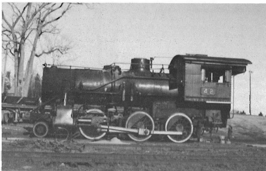
ABOVE AND OPPOSITE: The move of locomotive 42. November 19, 1991.
