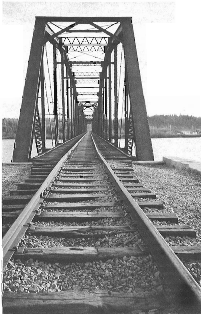
The CN Rail bridge over the Exploits River at Bishop's Falls, Newfoundland on November 14, 1990. This structure, about 927 feet long, was the longest bridge on the Newfoundland Railway. It is now used by pedestrians and all-terrain vehicles.
