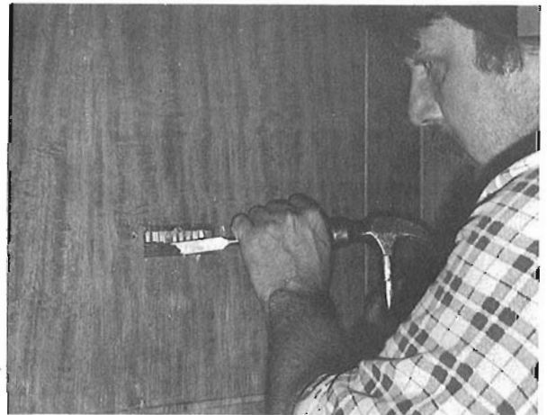
Veneer repairs. Project worker Peter Heather carefully removes a patch, which had carried a later light fitting, in preparation for setting in a new piece of matching Honduran mahogany. Taken in car "Somerset" on January 7, 1992.
