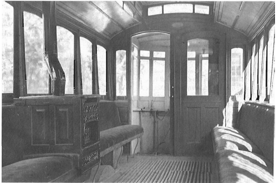
The interior of MSR 350 as seen on May 14, 1949. The interior of the car still has its original hundred year old paint finish and is little changed from the day in 1892 when it inaugurated Montreal's electric service. The double doors, which are the main feature of the "Accelerator" design, are clearly seen. Although the door (on the right in the photo) away from the platform steps was seldom used in Montreal service, loading and unloading was still faster because the entrance door was closer to the steps. Above the doors is an oval in which is inscribed the date, Nov. 3, 1891, of Brownell's patent. Note the coal stove used to provide heat in winter.
