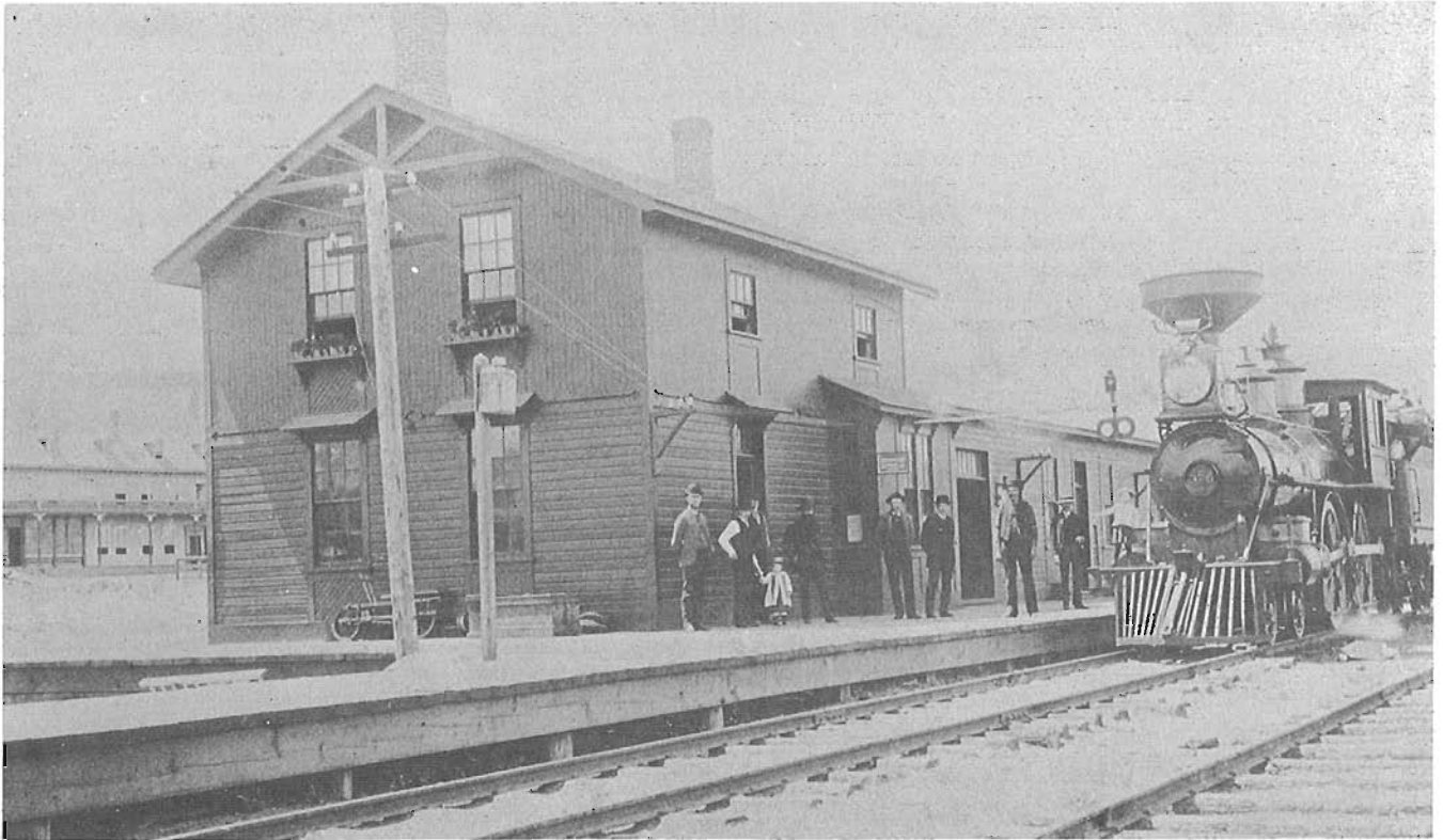
A circa 1890 view of Kamloops' first station with eastbound cpr train headed by 4-4-0 locomotive 376. Note velocipede below lower windows, window boxes in agent's quarters, disc type signal, lunch room to right and antlers fixed above loco headlight. At least one example of the disc signal survived elsewhere in Canada to 1957 or later.
