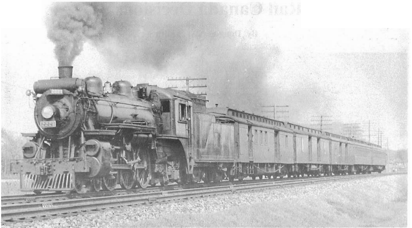
A magnificent view of CPR G1s class 4-6-2 No. 2221, built by MLW (construction number 49482) in 1911, hauling an all-wooden train, consisting of three head-end cars and two coaches, westbound through Pointe Claire, Que. in 1938.
