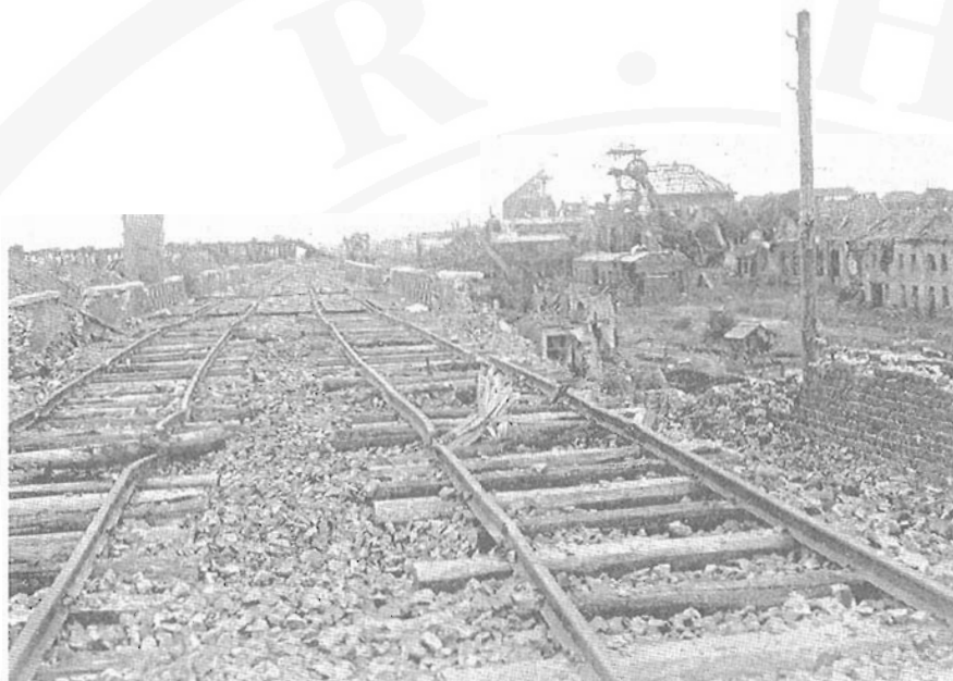
A section of badly shelled track on one of the standard-gauge lines in France. CRMW, January, 1919.
