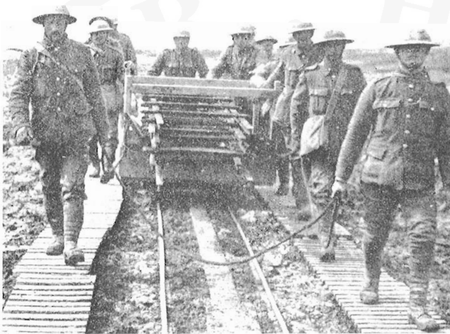
Moving supplies on a light railway recently laid over captured ground. The "duckboards", shown on both sides of the line, were necessary to avoid getting bogged down in the mud. CRMW, August, 1918.
