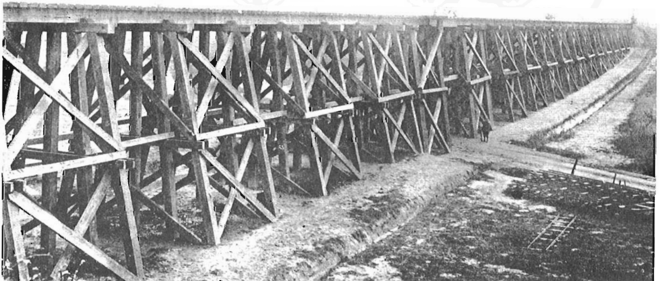
A trestle on the Frevent - Hesdin railway line in France. This trestle was 600 feet long, 40 feet high and contained 150,000 f.b.m. of timber. It was built by the Canadian Railway Troops in only 7 days. CRMW, August, 1919.
