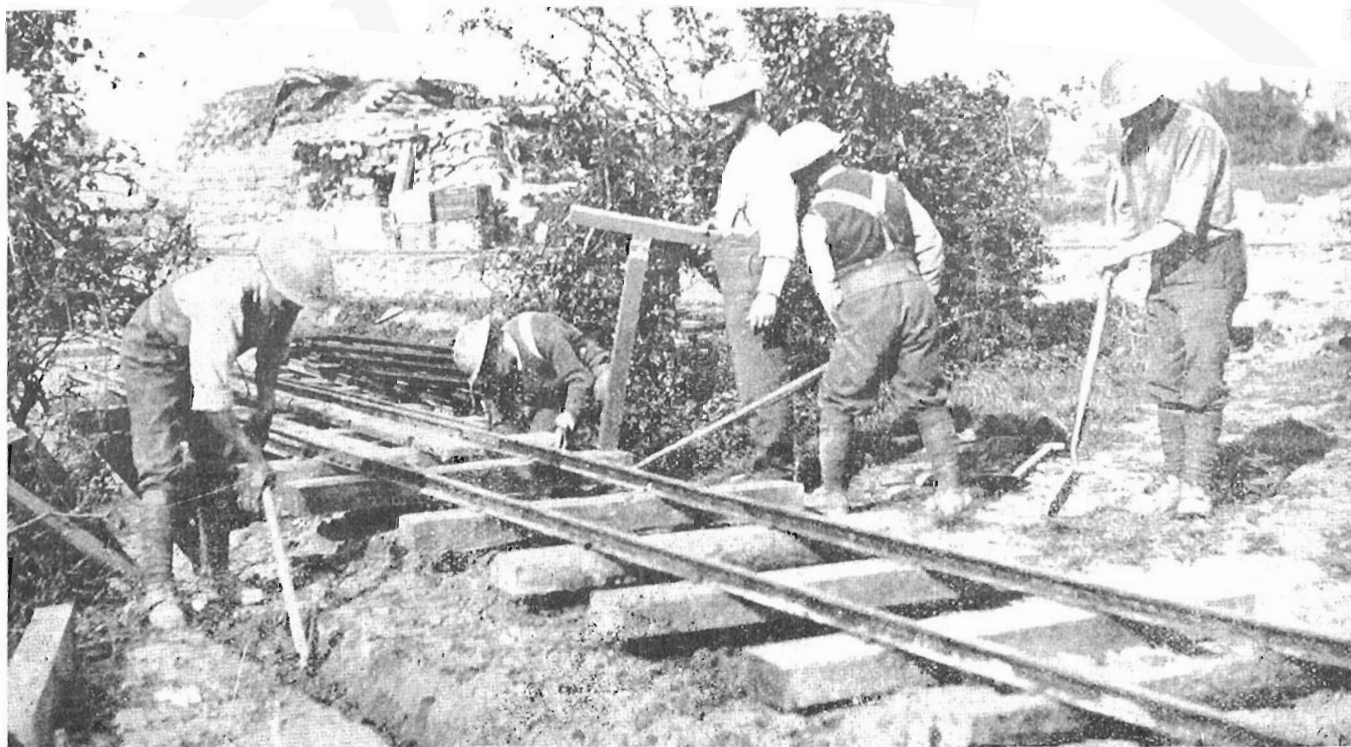
Members of the CORCC laying narrow-gauge track near the front lines. CRMW, August, 1918.
