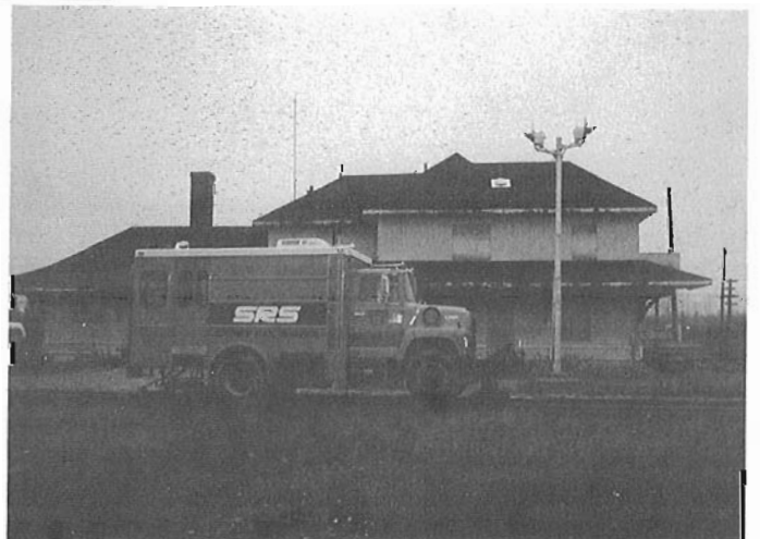
RIGHT: Early in the morning of October 26, 1993 SRS 805 is ready to start working north of Oba. The day is cloudy and dull as the crew prepare to depart. The station is boarded up and the hotel is in ruins. Oba is still an important freight transfer point between the ACR and CN, but the passengers who used to change trains here are long gone. However VIA Rail's "Canadian", as well as ACR 1 and 2, still pass this remote spot, far from any large city.
