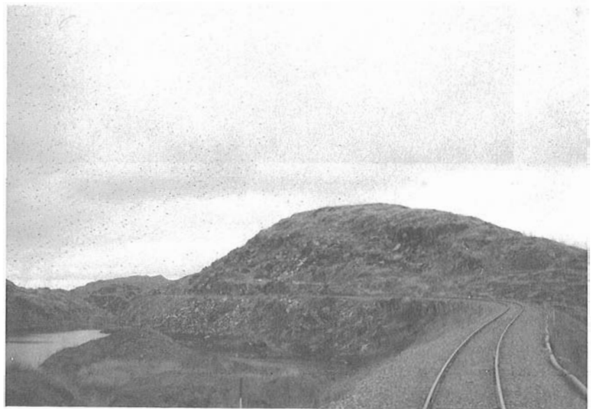
At mileage 17.3 of the Michipicoten Sub, the fire-damaged area is plainly visible.
