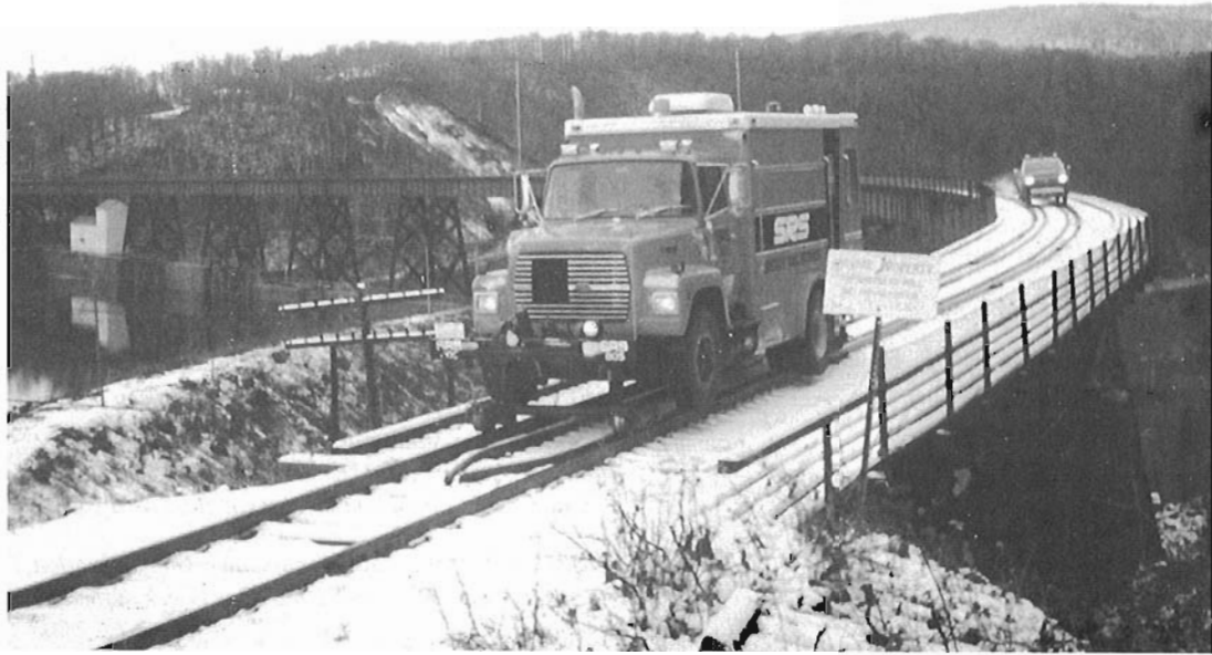
ABOVE: The most spectacular structure on the ACR is the Montreal River bridge. Since it is almost inaccessible by road, off-train photos of it are rare. Here, SRS 805 poses at the north end of the bridge on October 22. Near this spot the author spent the night and enjoyed a dinner of moose steak.
