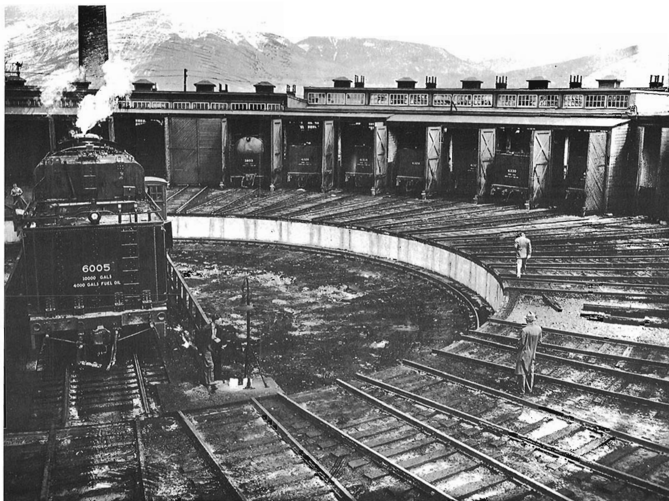
Another view showing the old, and part of the new, enginehouse at Jasper. Mountain-type locomotive 6005 is on the turntable, while most stalls are occupied. Engine numbers visible are 2-8-2 No. 3803, and 2-10-2's Nos. 4328, 4316, 4326, 4325, 4330.
