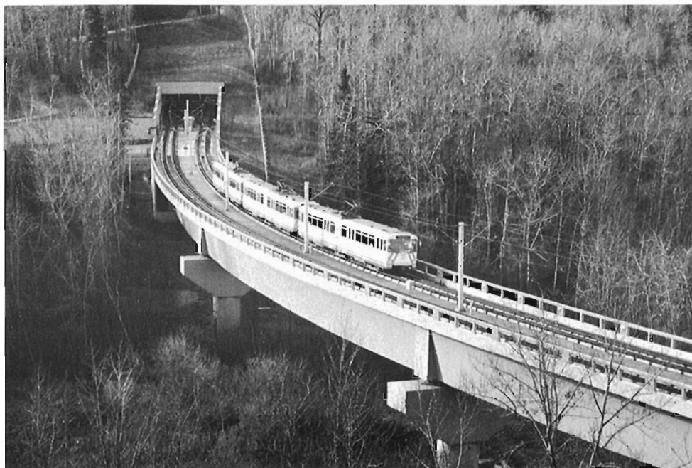
'Nephews' to unit #601 - a 6-car train of Edmonton Transit, northbound in November 1992 from University Station to Grandin Station, was approaching the tunnel of the north side of the North Saskatchewan River, running on the last section of the new LRT bridge which was built in 1991 and 1992. The train is composed of three 2-car articulated U2 units, built by Siemens-Duewag in Edmonton, Calgary and Germany. (George Duncan)
