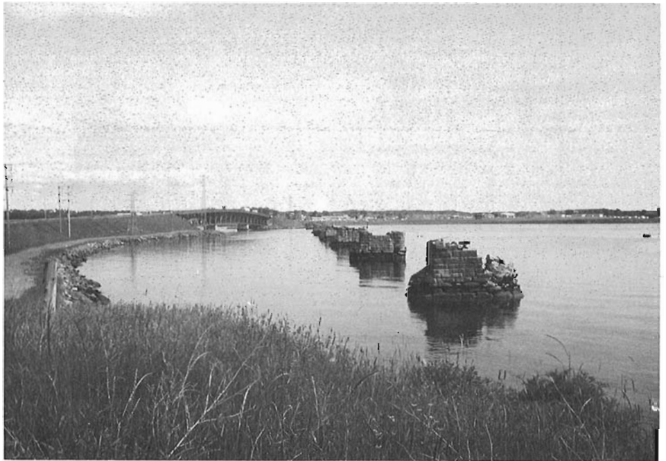
Remains of the Hillsborough Bridge piers at Charlottetown.
