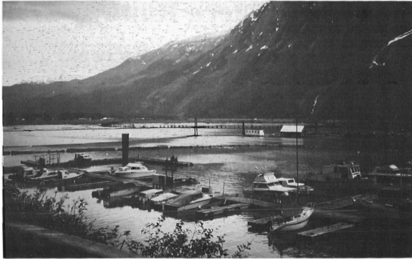
Stewart Bay, looking east from the Stewart - Hyder Road. The pilings that remain of the PCSLR trestle curve across this scene from the right toward the main land in the centre. June 1990. (M.T. Green)
