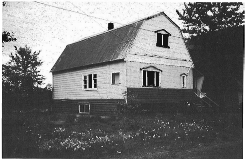
Private house on the east side of Railway Avenue in Stewart. Note the mansard roof covered in corrugated steel sections. June 1990. (M.T. Green)
