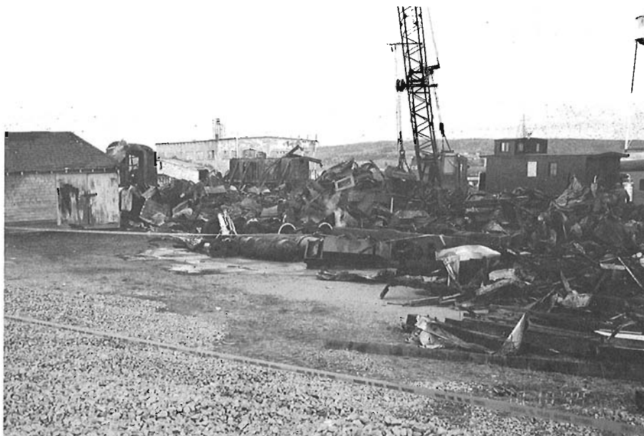
View of the ruins of the building, October 10, 1994.
