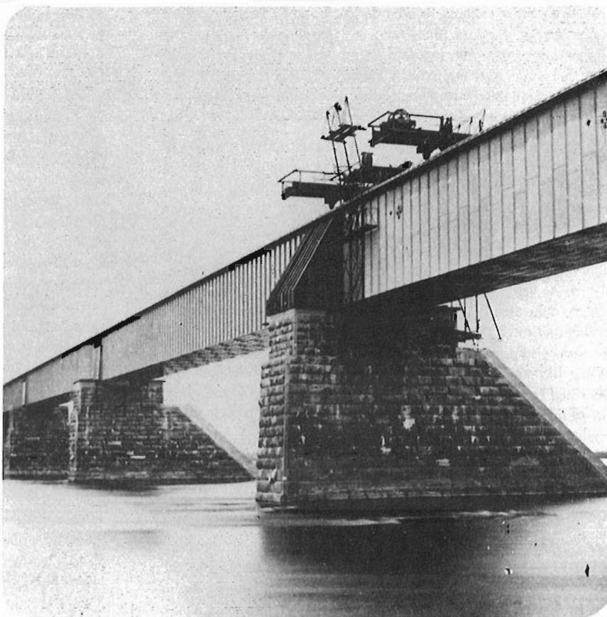
View from the north abutment on November 1, 1859. The great work was nearing completion. NPA photo No. 7010.
