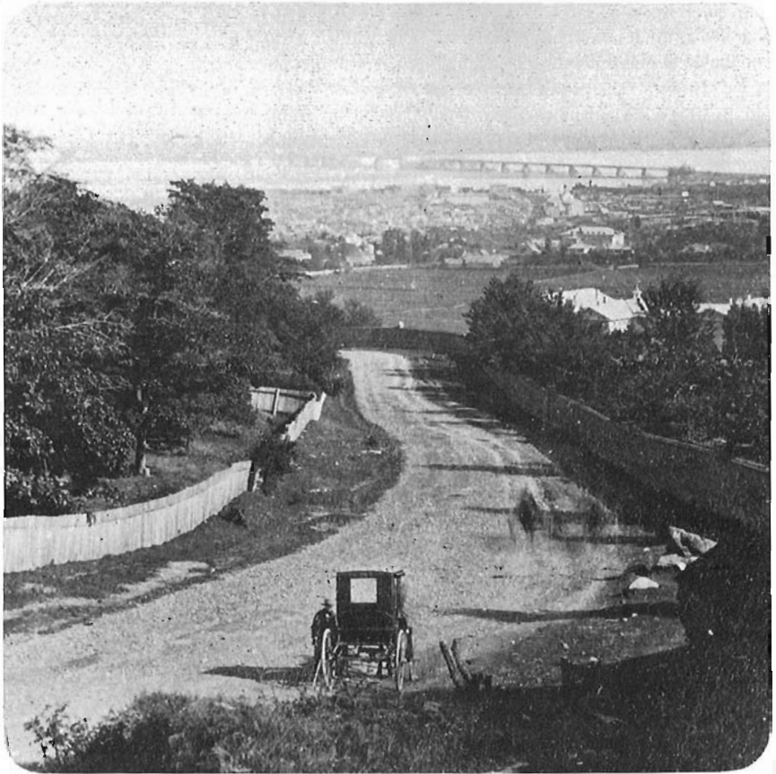
The work of construction of Victoria Bridge was visible from far away. This photo was taken looking down Côte des Neiges Road during the summer of 1859. The centre span is still unconnected to the others. The photographer's carriage is in the foreground. NPA photo No. 7097.
