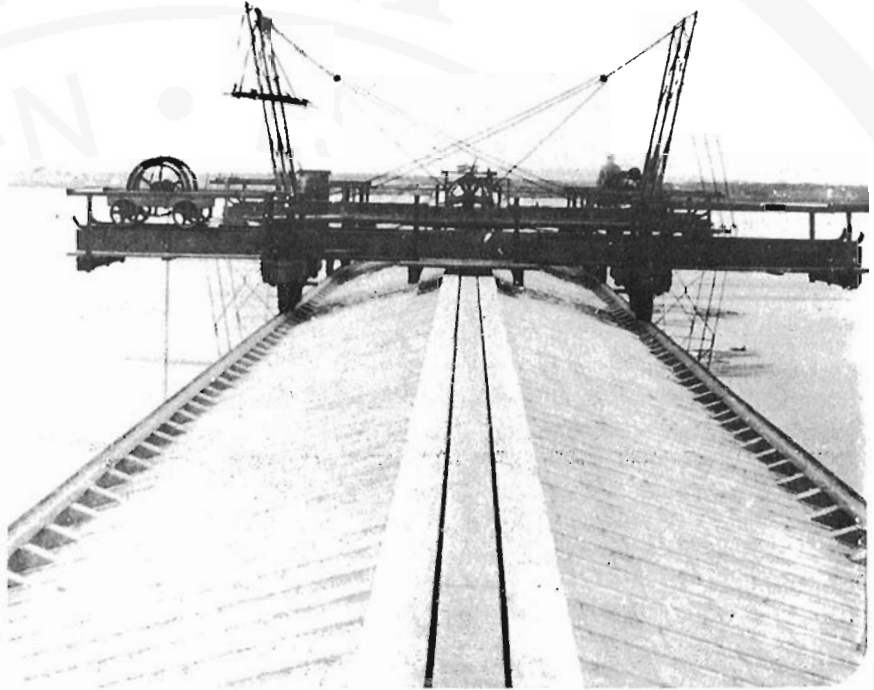
View along the top of the tube, in December, 1859, showing the roof walk as well as the "traveller" used for painting. At the time this photo was taken, the construction of the bridge was almost completed. NPA photo No. 7039.
