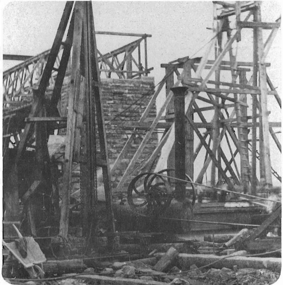
A floating derrick and pile driver at work in the summer of 1859. NPA photo No. 7015.
