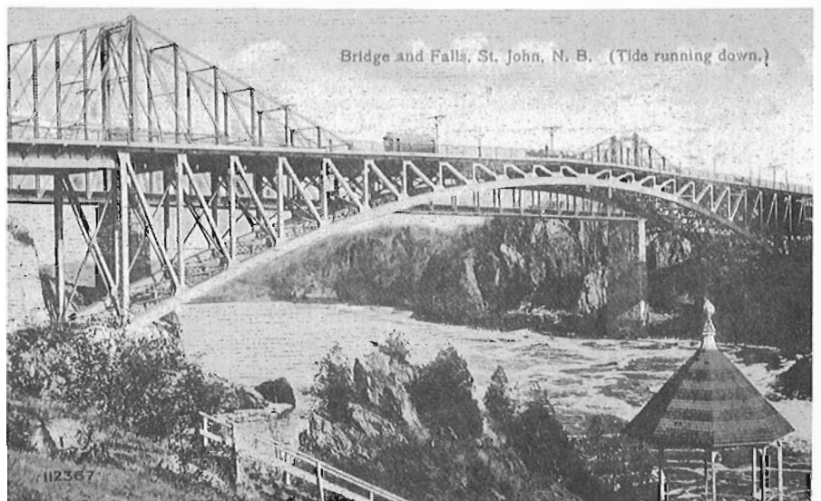
Two old postcards showing the bridges across the Reversing falls at Saint John. The top one was mailed in 1927, but bears a photo taken about 1921, just after the new railway bridge was completed, but before the 1884 cantilever bridge was torn down. The train is likely the early-afternoon departure for Montreal. The lower card, mailed in 1918, shows the old railway bridge, with the new highway bridge (and a Tillsonburg street car) in the foreground. The message reads "Saw this bridge from the train yesterday. Train passed over the bridge you see at other side of arch bridge. This is where the reversing falls are to be seen. St. John is as hilly as Sheffield, and nearly as smoky". Collection of Fred Angus.
