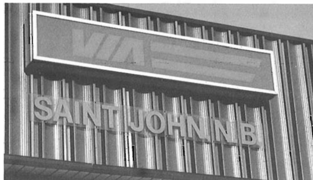
THIS PAGE AND OPPOSITE: Some scenes at VIA's brand new station at Saint John on the morning of December 13, 1994 as the second to last eastbound "Atlantic" stops. The station was in use for only a little more than a year.
