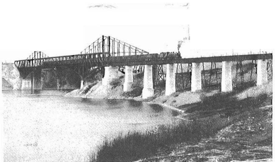
NEW C.P.R. BRIDGE OVER REVERSING FALLS, ST. JOHN, N.B.
