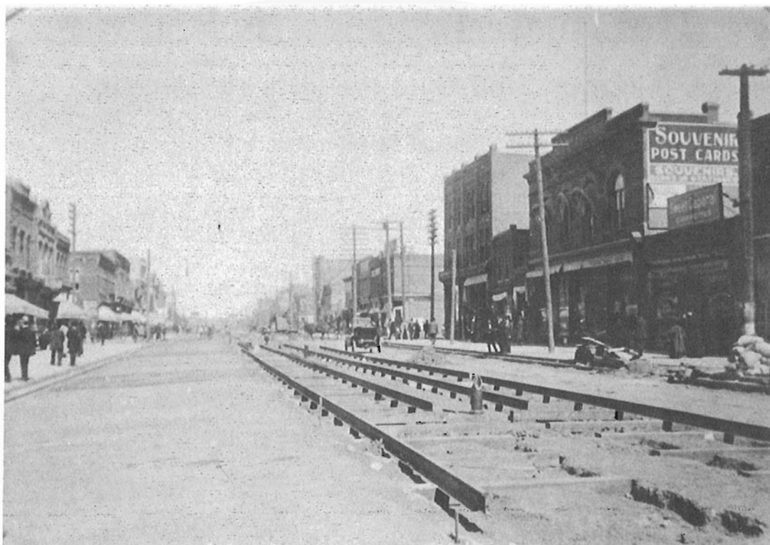
Tracklaying in progress on Main Street looking north, about 1911. Saskatchewan Archives photo No. R-A170.
