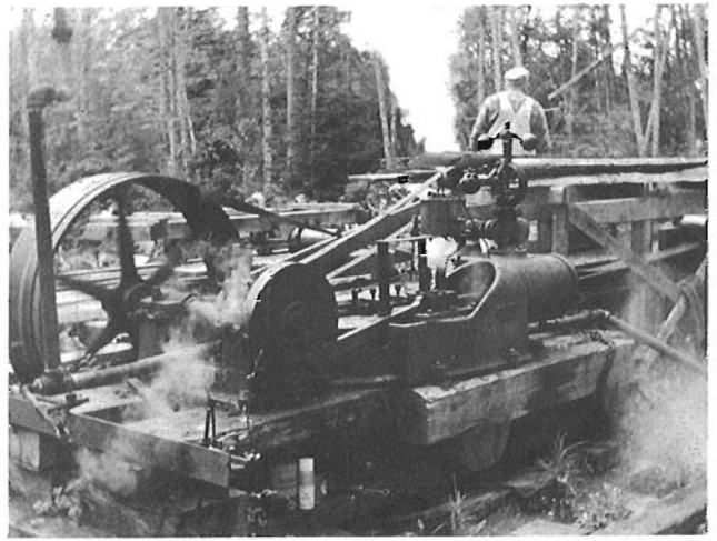
More steam operation at the Ladysmith Lumber Mill, June, 1980.
