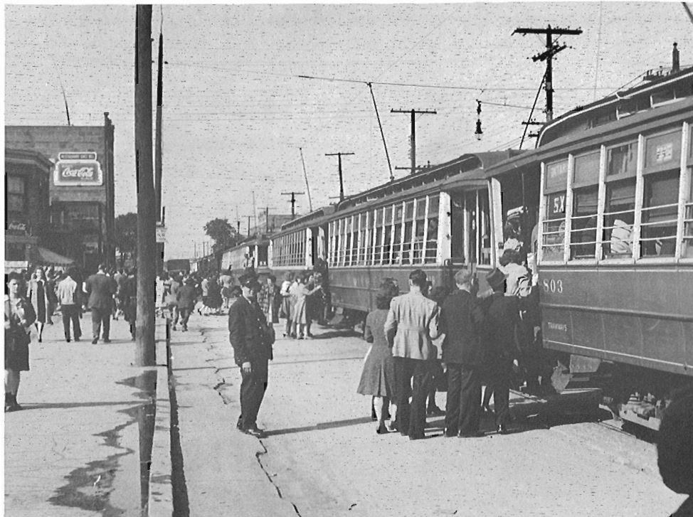
A long line of old Montreal streetcars waits on Ontario Street East, in the summer of 1943, as workers from the war plants prepare to board. All these large cars were built between 1906 and 1908, and some had been retired, and slated for the scrap pile, in the 1930s. Reconditioned and returned to service, they did great work during the war. CRHA Archives, Binns collection.
