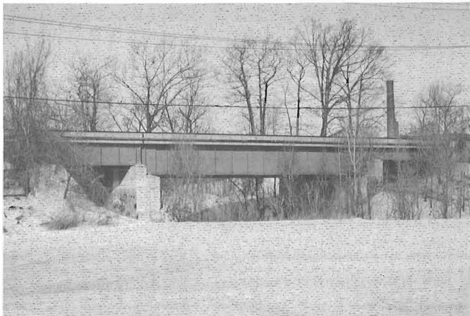
Mimico Creek bridge. The left span of the Mimico Creek trestle is where the Toronto Suburban once had a subway under the mainline of the CPR between 1917 and 1935. The spans closest were added in 1913 when this right-of-way was double tracked. Islington Station was a quarter mile to the left of the photo.
