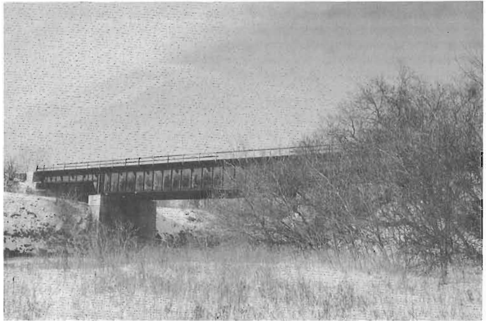
Etobicoke River Trestle and Original Pier
