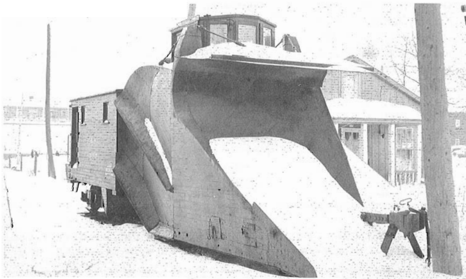
LEFT: Snow plow 307 had come from the CNR in 1940. Built by Russell in 1917, it did not have any electric equipment. This photo was taken at Granby in January, 1951.
