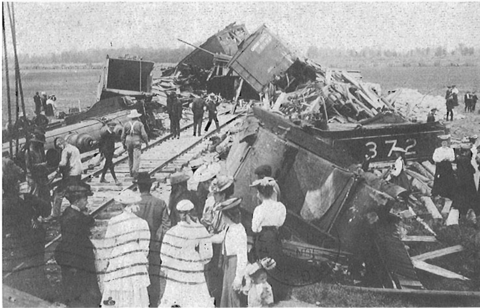
The best show in town. The wreck occurred about a mile and a half from Fergus, and it attracted quite a crowd in the pleasant June weather of 1906. This view looks north. Note the light 56 lb. rail. At the right, cleanup crews have piled intact bags of flour or cement for salvage. Workers are moving debris to the side: reopening the track was the first priority.
