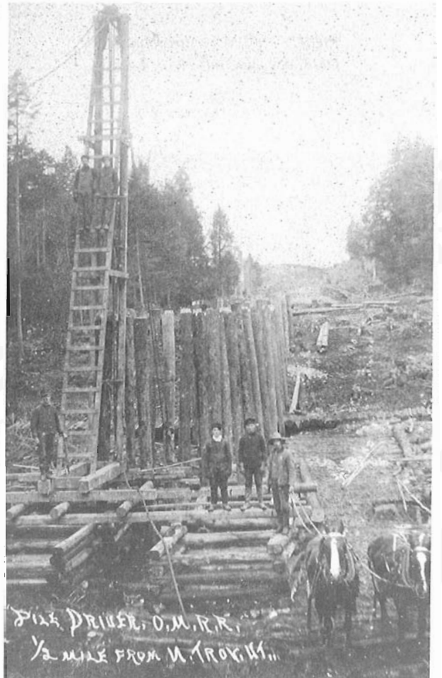
Pile driver, OMR, 1/2 mile from North Troy, Vt.
