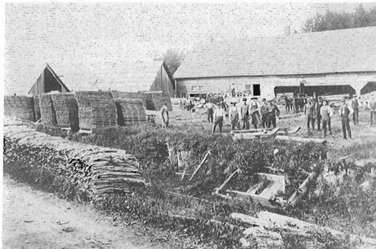
Lumber mill beside the OMR tracks.
