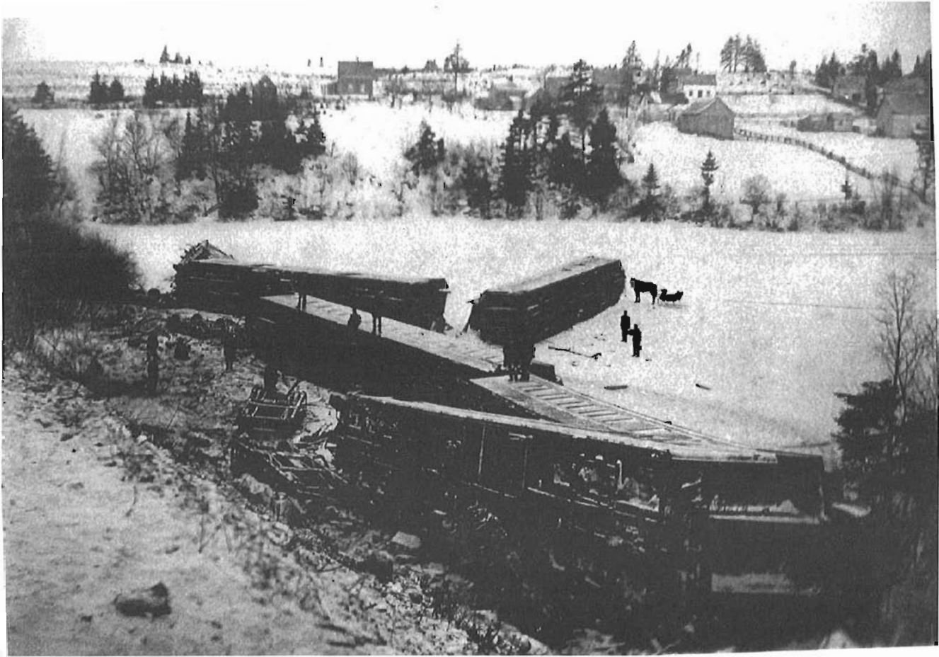
Looking down on the wreck from the railway right of way. The sleeping car "Sherbrooke" is nearest to the camera. This car was destined to serve the CPR for another 65 years before being preserved. Photo courtesy of the Keillor House Museum, Dorchester N.B.
