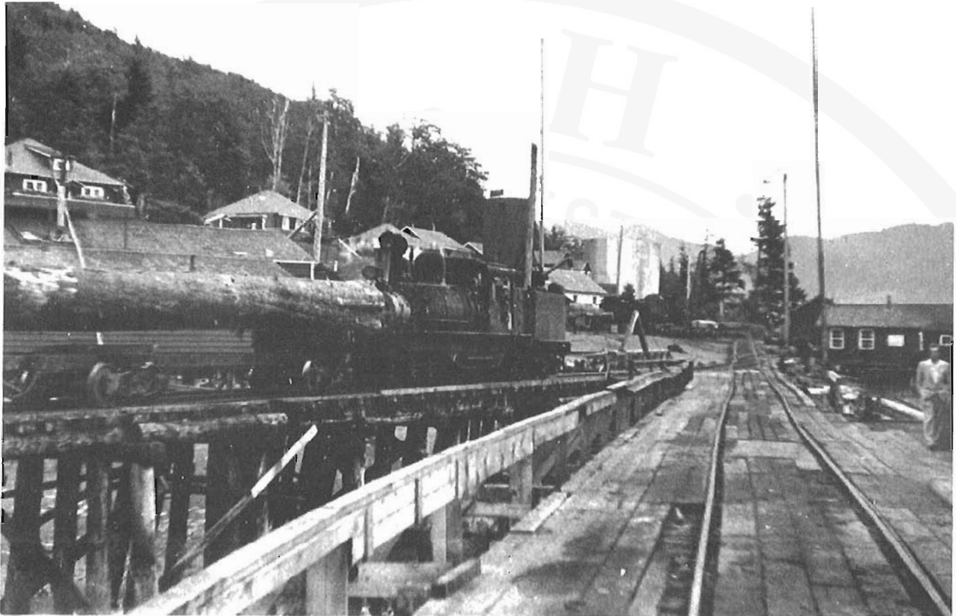
The last loads of logs being brought down to the dump by Shay No. 1 on August 31, 1955. Note that the long log ahead of the locomotive is spanned across two skeleton logcars. -MacMillan Bloedel Collection
