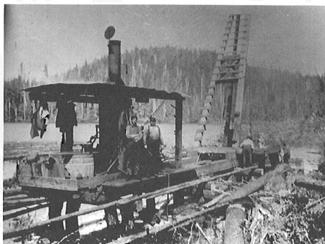
A pile-driver was useful in extending the trackwork through the marshy areas being logged. This view is probably along the shore of Skidegate Lake. -Stan Unsworth photo, Author's collection
