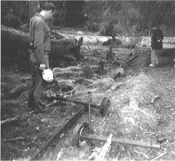
The tramway used to haul copper ore from the IKEDA BAY MINE was 3-foot gauge. These photos of the remains of the frame of one of the ore cars gives an idea of the load that the horse pulled from mine to dock.
