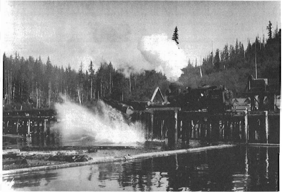
A.P. Allison's Climax No. 2 at the Cumshewa Inlet log dump in 1938. The locomotives were coal-burners at this time. The coaling platform is just to the right of the locomotive. -B.C. Forest Service, 5328
