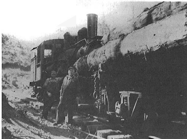
Allison's Climax No. 1 during the early years of the logging railway at Cumshewa Inlet. The track is unballasted and light rail was used. -Stan Unsworth photo, Author's collection
