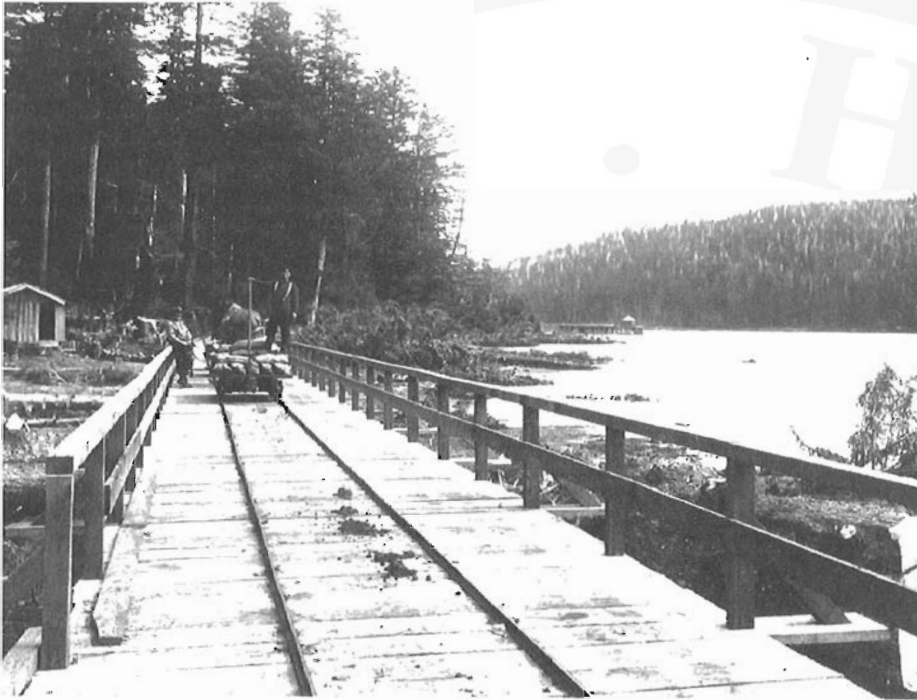
The Ikeda Mines tramway along the shore. The horse-drawn tramway car is loaded with sacked ore. In the distance is the steamer dock. BC Archives & Records Service, H-04581
