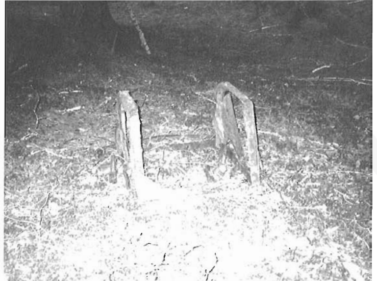
The tramway used to haul copper ore from the IKEDA BAY MINE was 3-foot gauge. These photos of the remains of the frame of one of the ore cars gives an idea of the load that the horse pulled from mine to dock.
