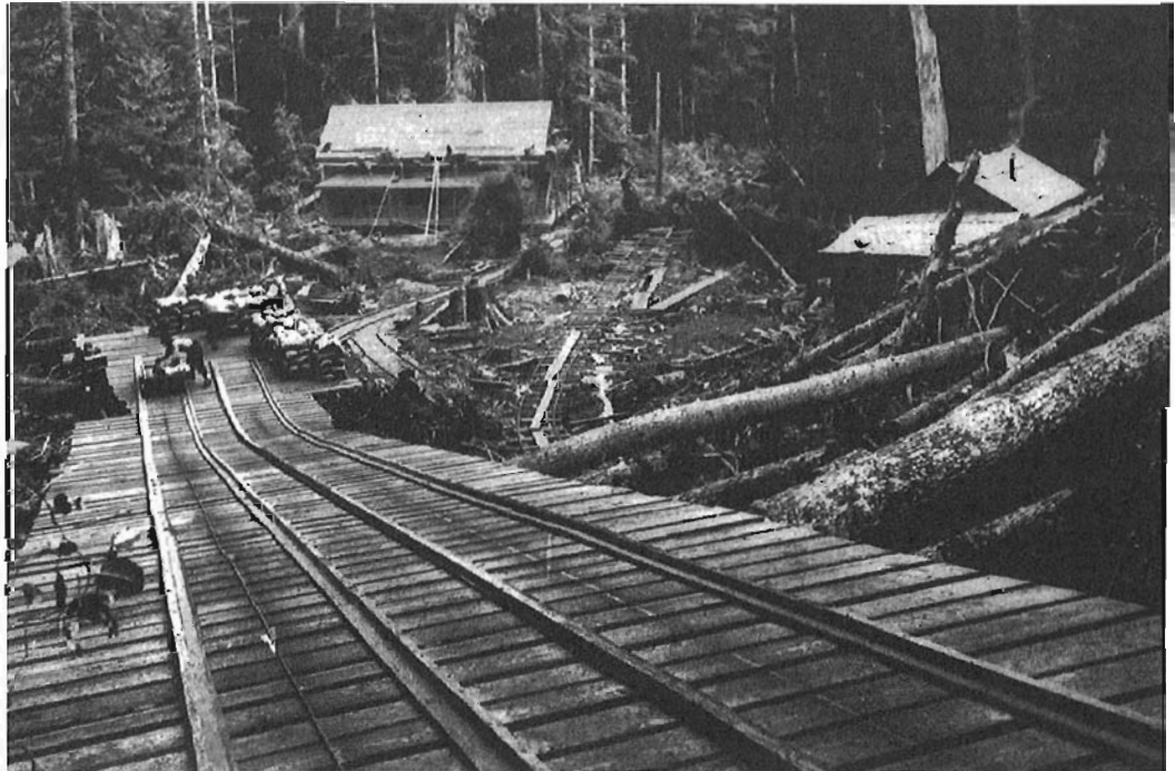
The Ikeda Mines on Moresby Island during the construction of the camp buildings probably in 1907-08. The view is from the upper tunnel. In the foreground is the wooden-tracked incline system used to transport sacked ore. Note the tramway trackage beyond the ore. -BC Archives & Records Service, H-04582
