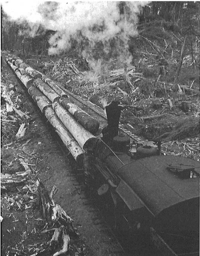
The big Heisler was No. 3 on Allison's operation. These two views show the engine, with a cut of eight logcars, backing down to the log dump in July 1940. -H.W. Weatherby photos, B.C. Forest Service, 2447/28 and 2483/9.
