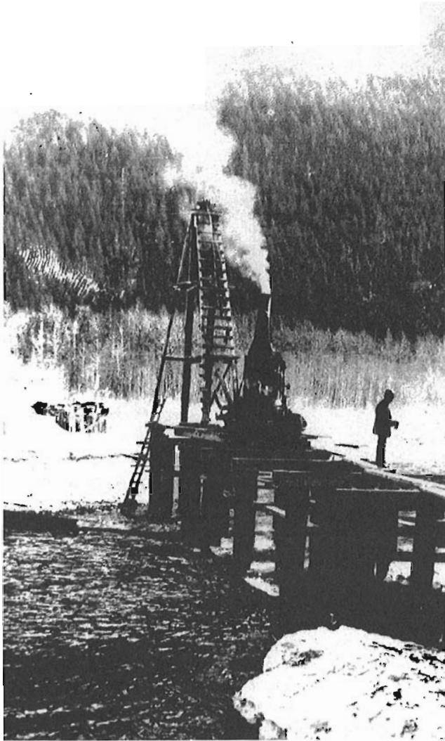
No. 72764 - CNER, about April 10, when the pile-driver had reached across the first main channel of the Bear River, but no ladder could reach across to the first gravel bar. The contractor, Ernie Workman studied the current below the bridge on the down-river side of the bridge
