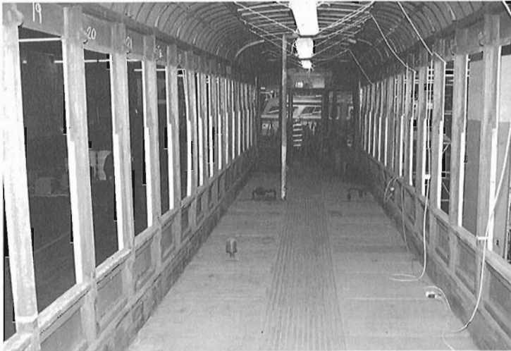
Rebuilding the structure, interior view. Photo courtesy Bill Bailey.
