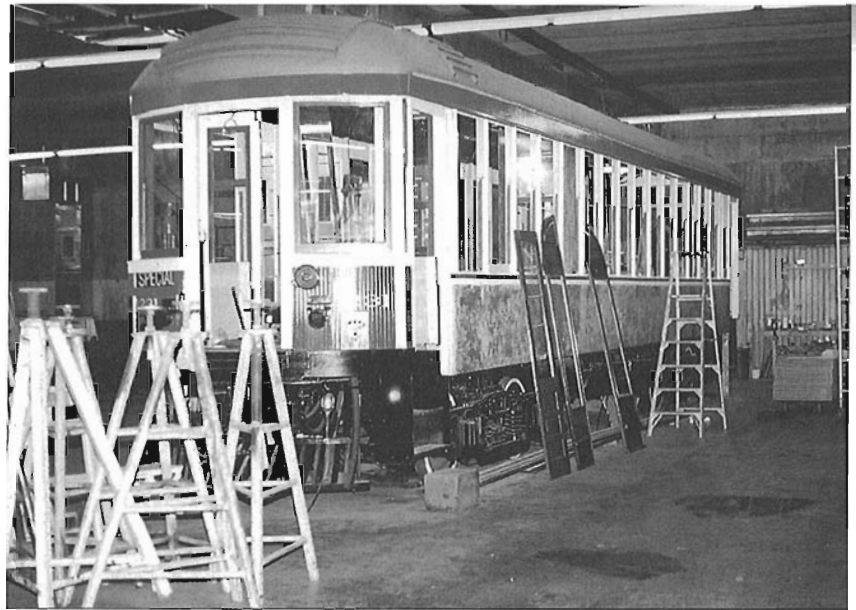
Pardon the debris, but this is 1231 in July, 1997, note the motorman's door and smoking section bulkheads leaning on the side of the car.
