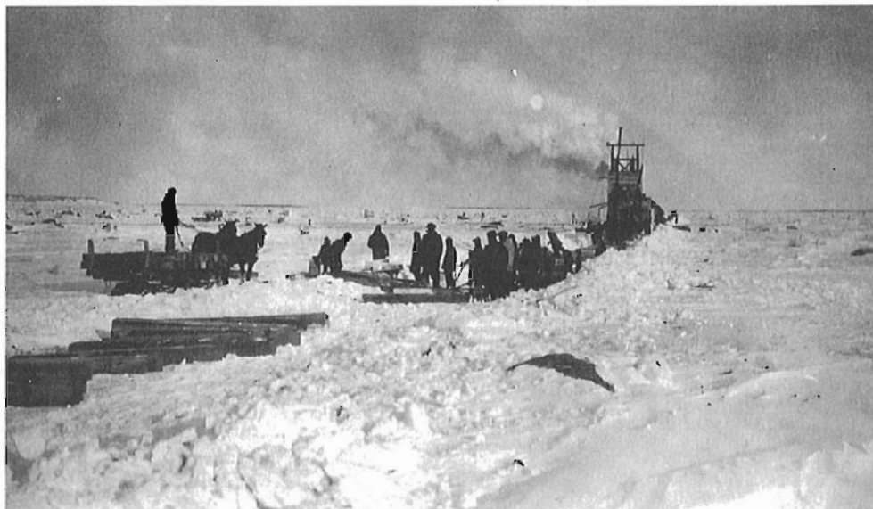
Laying track in the snow; April 1, 1929.
