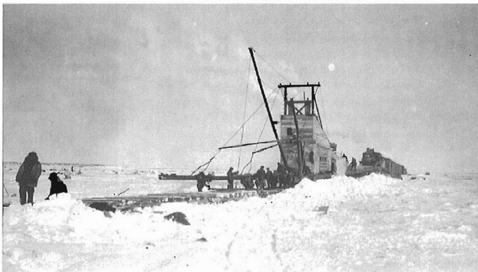
“Pioneer” laying track at Mile 510 on the Churchill line; April 1, 1929.
