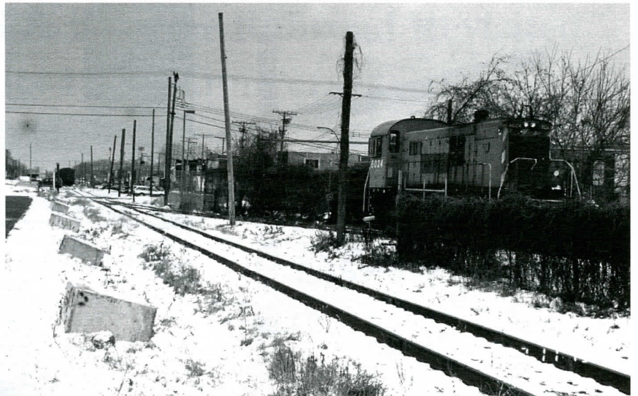
RIGHT: Former CPR 8024 switching at Canadian Allied Diesel.
