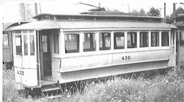
ABOVE AND LEFT: A rare comparison of the largest city cars to operate in Montreal before 1900 as they appeared at the beginning and end of their careers. These were the four members of lot 13, built by Ottawa in 1895. Above, left we have one of the few Ottawa Car Co. builder's photos to survive, number 436 as built. Directly above we see 432 as it appeared in 1948 as a salt car. Of this lot, 430 was destroyed in the fire of 1898.
