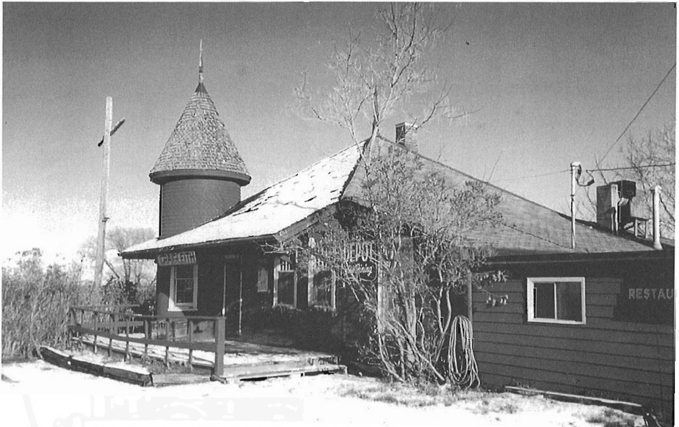
External view of station, looking south. It is on its original site, but has been turned 90 degrees from its former orientation.
