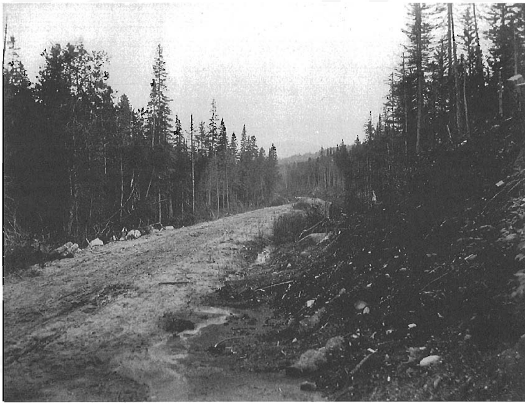
GRADING ON INTERNATIONAL RAILWAY MEGANTIC.
