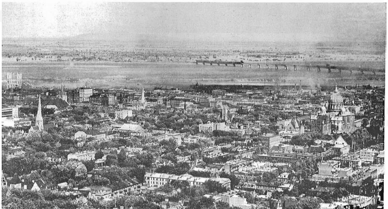
Montreal from the lookout on Mount Royal during the rebuilding of Victoria Bridge. The progress of the work dates this photo to mid June, 1898. In the middle foreground is the Prince of Wales Terrace, named for the prince who officially inaugurated the original bridge. This historic terrace was torn down in 1971
