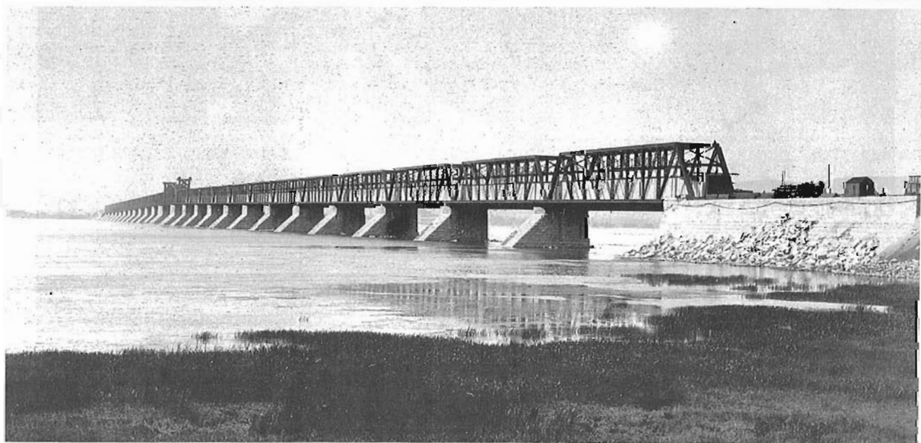
Another month's progress is depicted in these three photographs. In the top view, July 18 1898, all spans but the centre one are built. The middle photo, July 24 1898, is a more detailed view as work on the spans paused awaiting the delivery of the steel. By August 18 1898, lower photo, the new centre span was in place. National Archives of Canada, Photos PA-202517, PA-202509, PA-202518.
