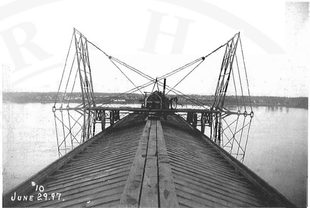
The "traveller" running along the top of the old bridge on June 29, 1897 (nine days after Queen Victoria's Diamond Jubilee). National Archives of Canada, photo No. PA-202499.
