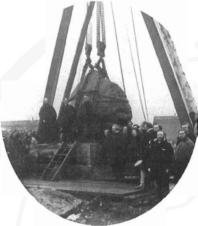
Putting the "Irish Stone" in place, 1859.
