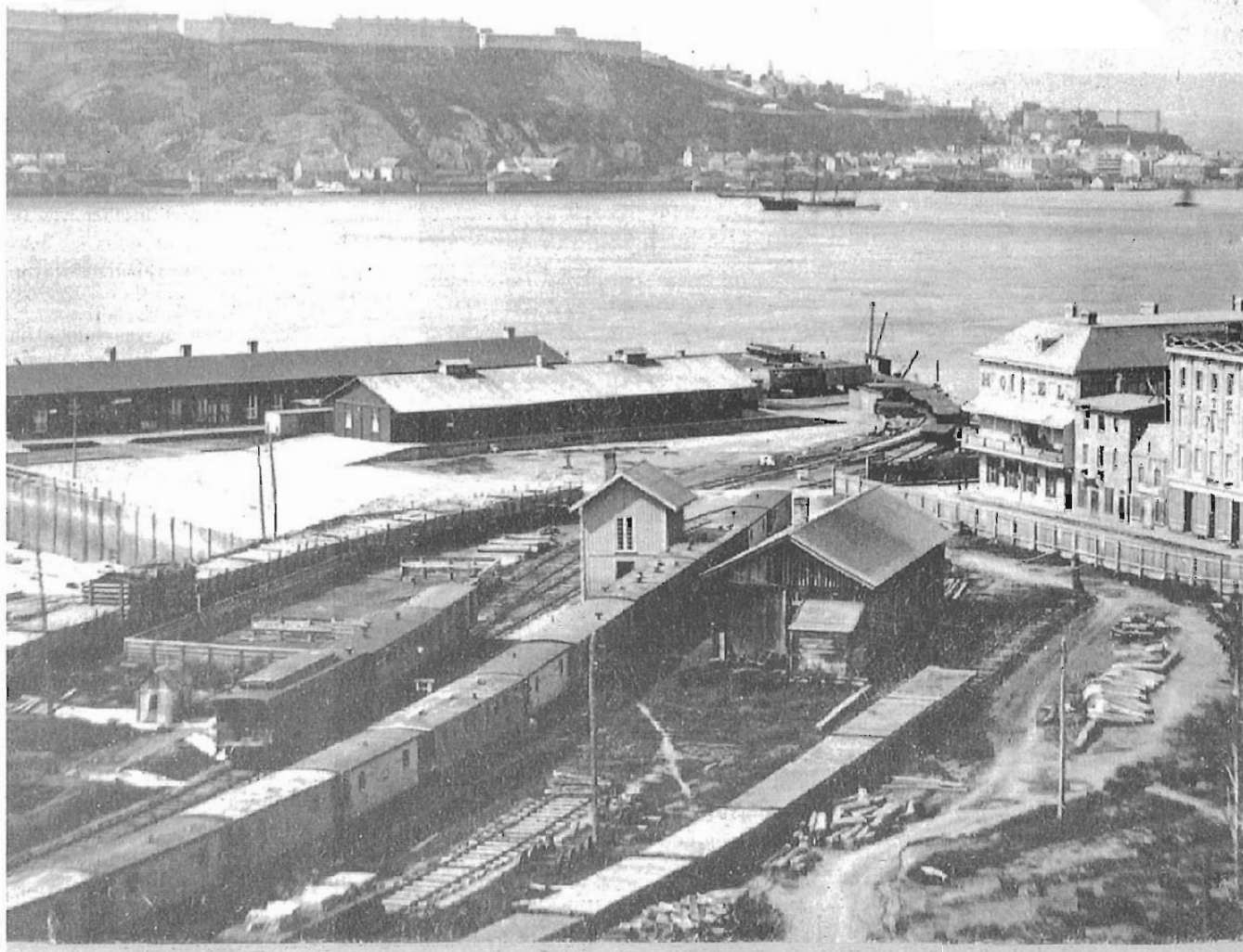
A view of the docks and terminal at Point Levi about 1864. In the background is Quebec City and the Citadel. In the left foreground is a train of the infamous immigrant cars; clearly just boxcars with windows cut in the sides. What a contrast to the regular coach, with an early clerestory roof, seen on the adjacent track. This is one of the few photos extant that show the immigrant cars. It is from a stereo view published G.R. Proctor of Salem, Massachusetts. National Archives of Canada, photo No. PA-143770.
