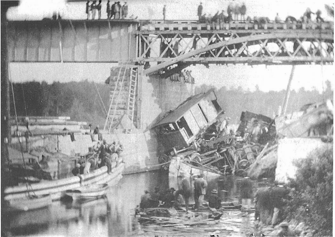
This photo of the wreckage is one of three taken soon after the accident, probably on June 29. It differs from the photo on the cover in that it is in horizontal format and there is no train crossing the bridge. The brake van, the last to fall, is scarcely damaged at all. National Archives of Canada, photo No. C-3285.
