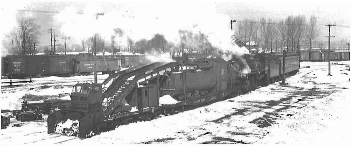
ABOVE: This snow melter was photographed in action in February, 1948. It was useful in yards where there was little room to dump the snow. Canadian Pacific photo No. 12418.
