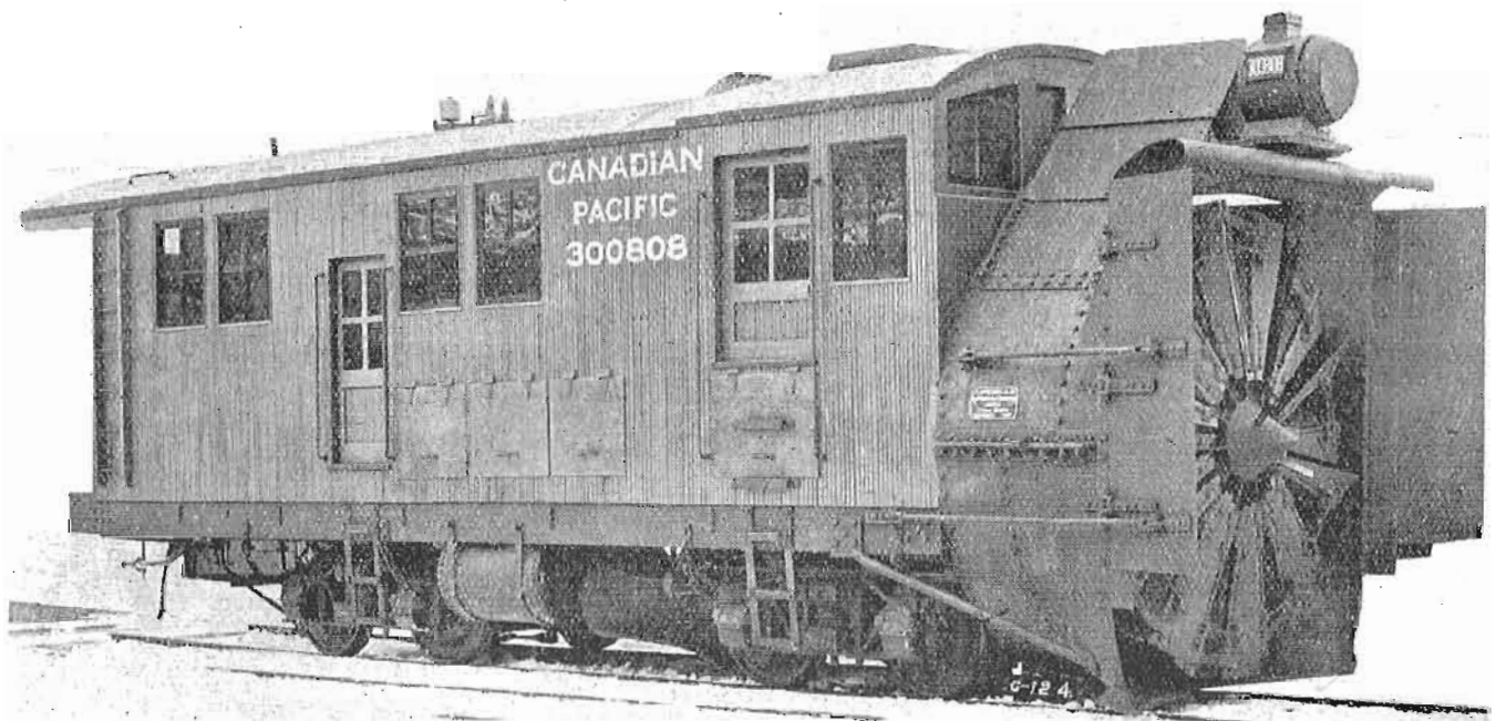
Fig. 31. Canadian Pacific rotary snow plough, built in 1907.
