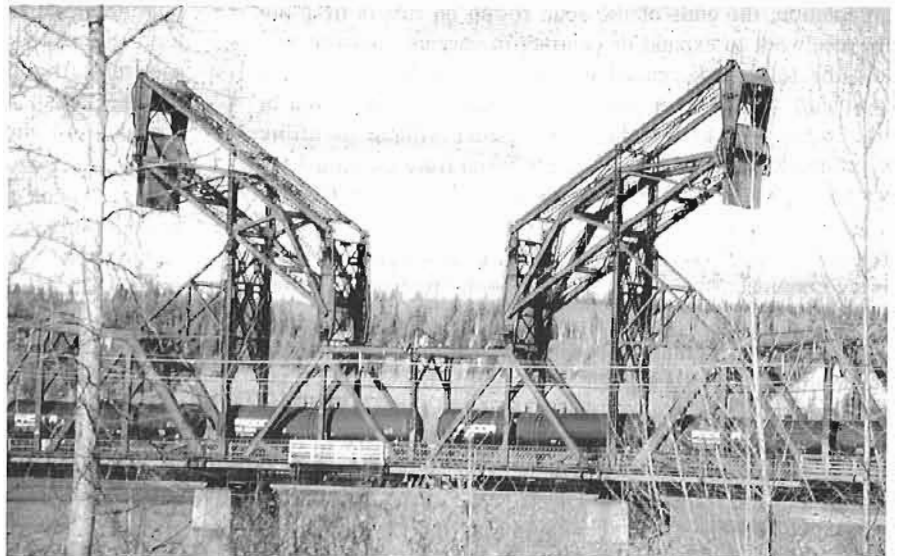
Design details of the lifting span which has been secured shut since 1954. Photo by author.
