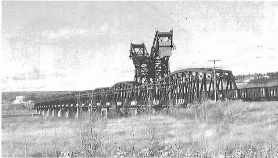
View of bridge from east bank in October, 1999. Note the loaded coal train passing over it. Photo by author.
