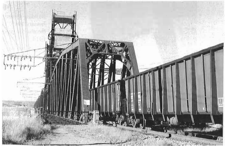
The eastern end of the bridge carrying a loaded coal train bound for Prince Rupert, in October 1999. Photo by the author.
