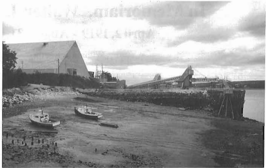
RIGHT: Low tide at Hantsport, on the south side of the Avon River, showing Fundy Gypsum's storage shed and loading pier. Ocean-going ships will not be able to approach the pier to load until 3 hours before high tide.
