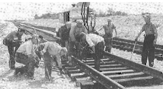
CNR crews laying the new track between Cornwall and Brockville, 1957
